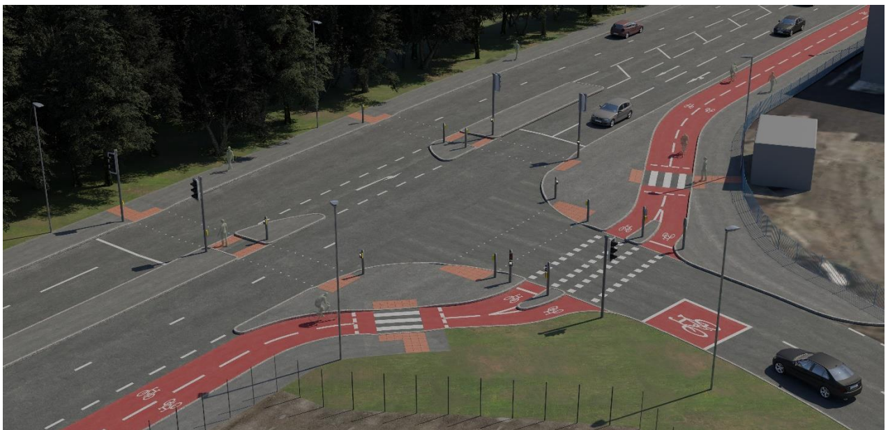
Figure 3: Proposed modifications and upgrades at the junction of John Gilbert Way and Wharfside Way including separate signal-controlled crossing facilities for both cyclists and pedestrians.
