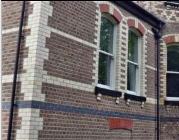
Photograph 10: Polychromatic Brickwork and Header Bond
