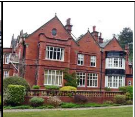
Photograph 89: Victorian Property with Decorative String Courses and Hood Moulds, Charcoal Road
