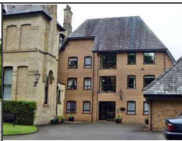
Photograph 134: Extension to Inglewood, St Margaret's Road
