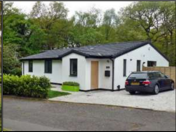
Photograph 97: Modern Bungalow, Next to the Reservoir
