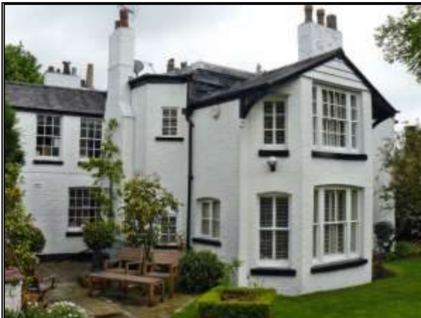
Photograph 12: Painted Brickwork, Parkfield Woodville Road
