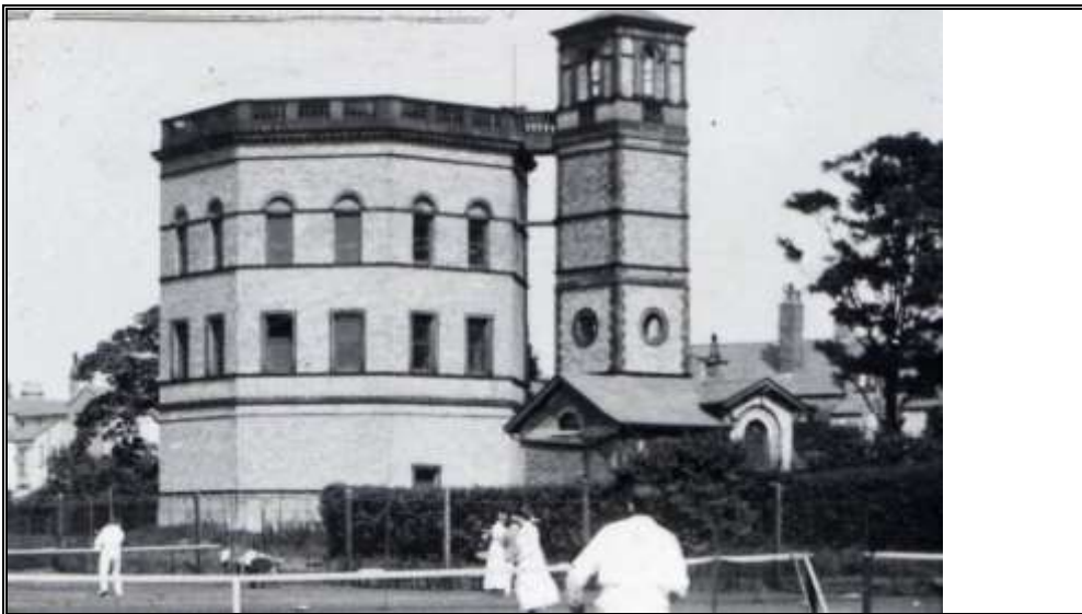
Photograph 5: Water Reservoir and Tower with Bowdon Lawn Tennis Club in Foreground. (Altrincham Area Image Archive, BM 0414)
