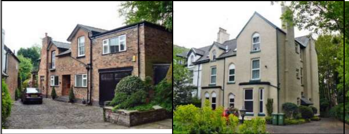
Photograph 14: UPVC Replacement Windows to Grove Cottage
