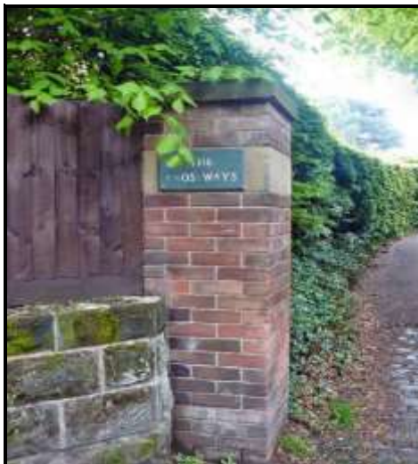
Photograph 123: Modern Replacement Gate Post, St Margaret's Road
