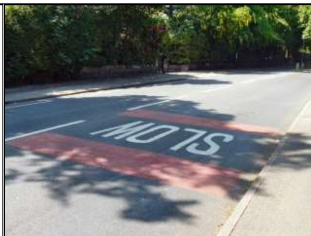
Photograph 128: Inappropriate Road Markings, Park Road
