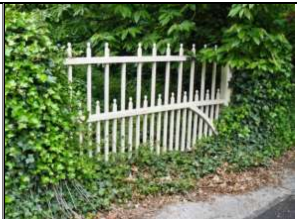
Photograph 51: Gate and Gateposts (under Ivy) of Former Carriageway
