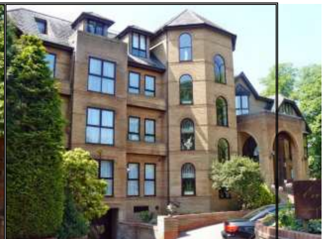
Photograph 71: Apartment Building Green Walk
