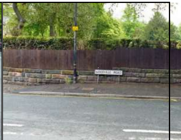
Photograph 29: Stone Wall with Fencing Above, Woodhale Road
