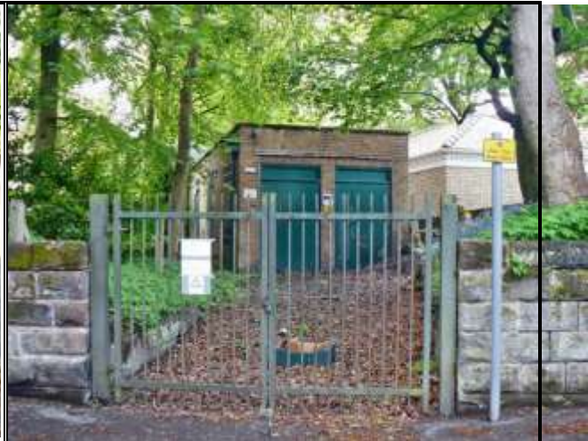
Photograph 27: Electricity Substation, Booth Road
