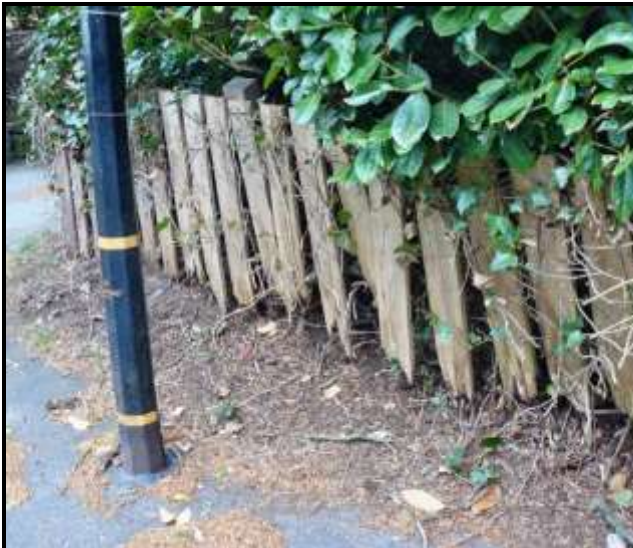
Photograph 121: Timber Fence along Charcoal Road
