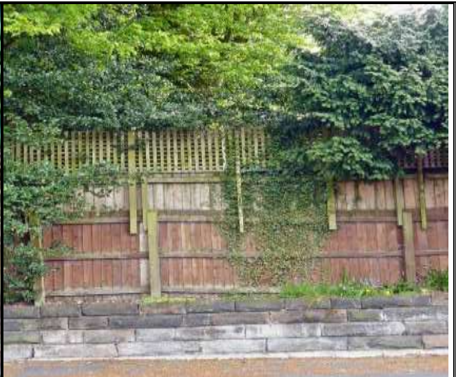
Photograph 122: Inappropriate Boundary Treatment along Oldfield Road
