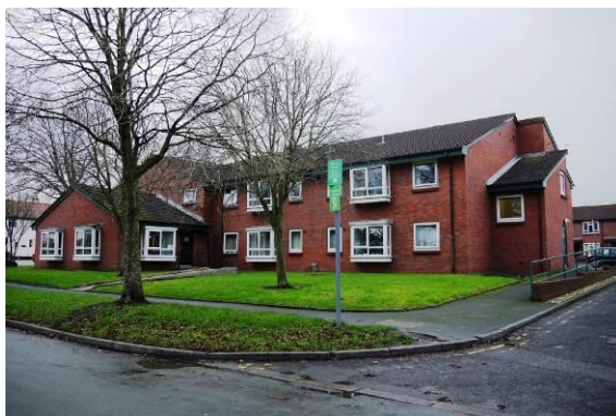
Modern development outside the Conservation Area
