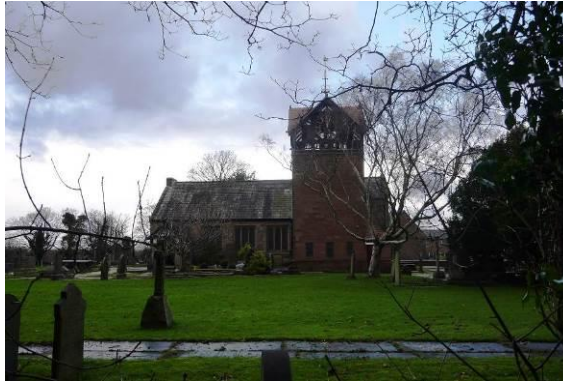
View of the church, south elevation
