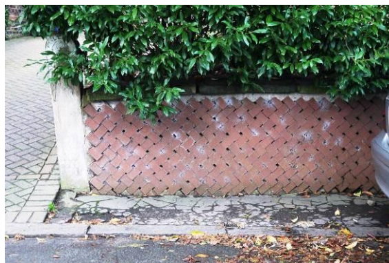
Boundary treatments along Church Lane
