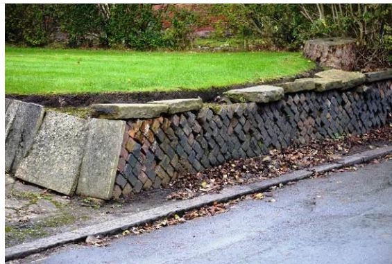
Boundary treatments along Church Lane
