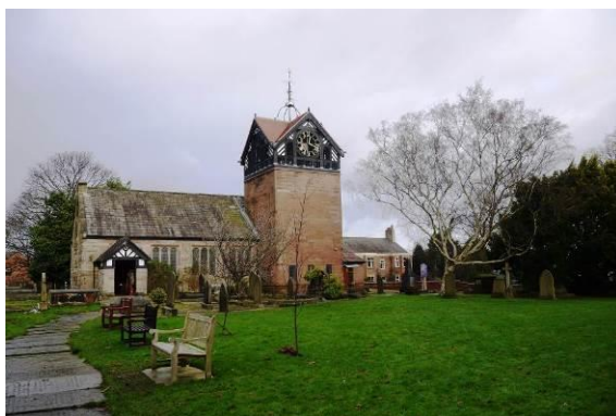
View of the church, south elevation
