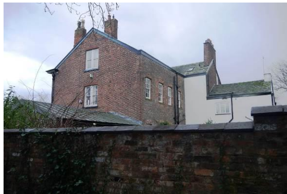
The rear of Ashton New Hall
