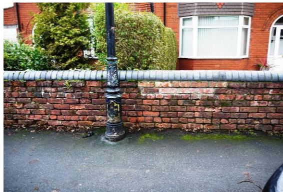
Boundary treatments along Church Lane
