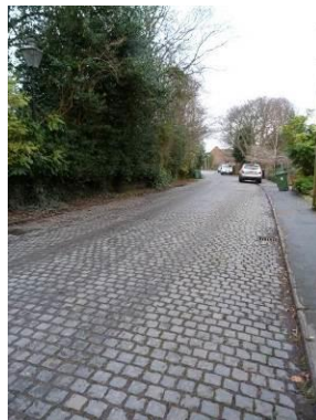
Road surfacing within the character zone
