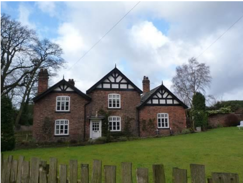
101 Woodhouse Lane - side elevation
