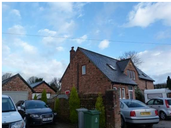
Characteristic large gable dormer recreated at The Brambles, Church Green
