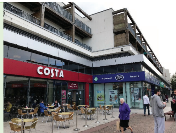
Figure 2: Eden Square Commercial Units
