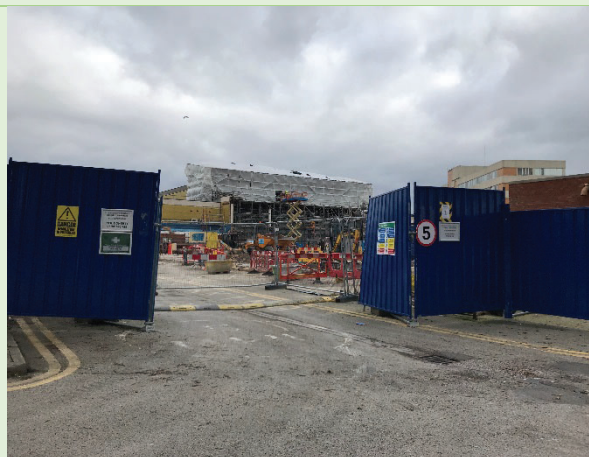
Figure 3: Demolition site adjacent to the mall
