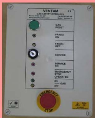
The interlock will shut off the gas supply to these appliances if there is inadequate air movement.
