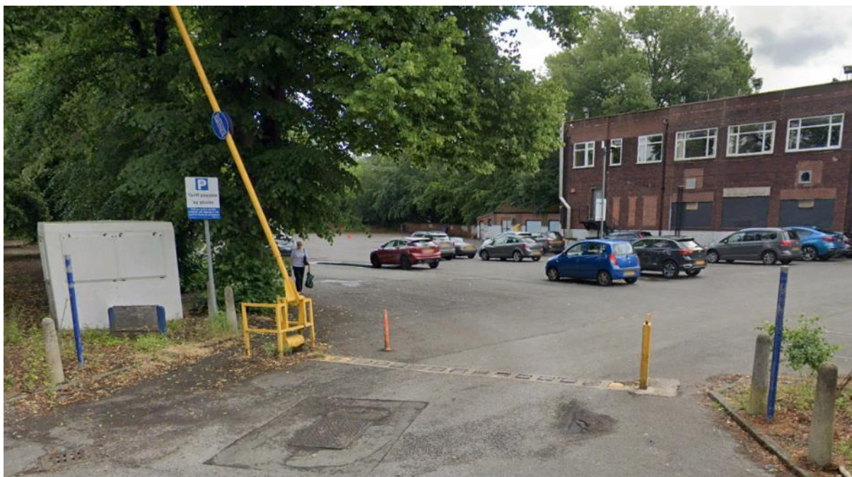
Figure 1. The entrance to the Mecca Bingo carpark with security barrier, concrete bollards, sub station and open carpark area
