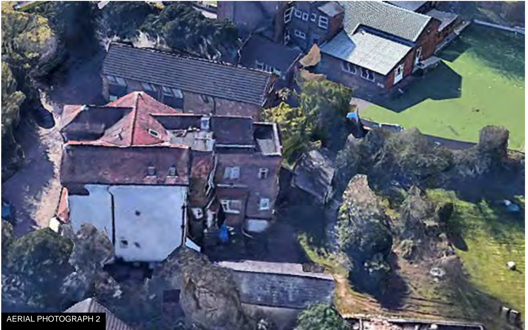
From the north the extent of alterations and extensions to the rear again show the detrimental effect of adaptation. The north flank of the original building is rendered white and almost blank.
