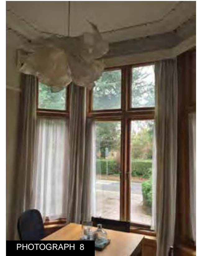
One of the two original main reception rooms (to the RH side of the front door on entering) with original ornate cornice over the tall windows. The rear of both rooms have been truncated (see current floor Plan) to provide galley kitchens.
