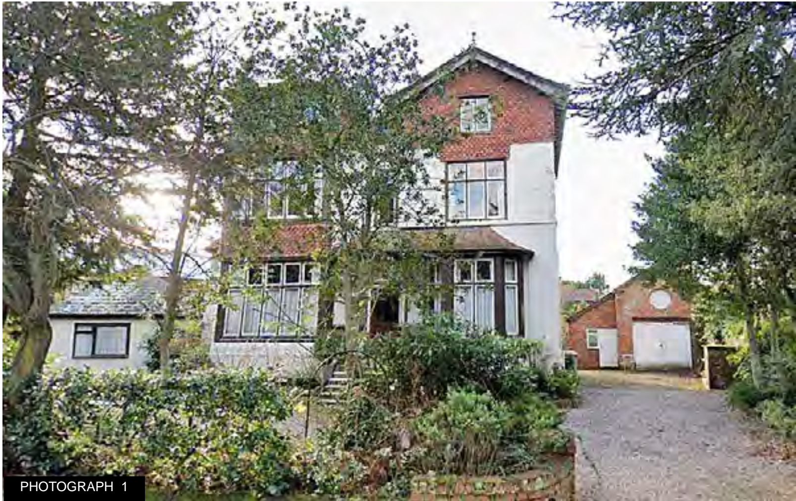
The front (east) elevation facing Oakfield. This is the one face of the building (including the porch) that appears to be original and largely intact. This elevation is assymetrical and the LH wing in particular has a very large area of window openings for a building of this age.
