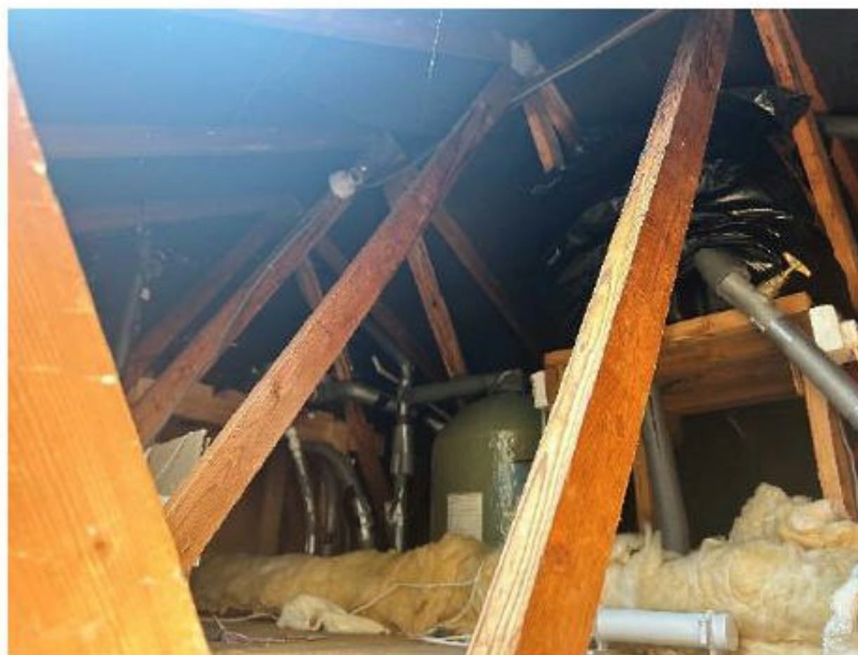
Plate 1 - Loft void within western section of Building 2.
