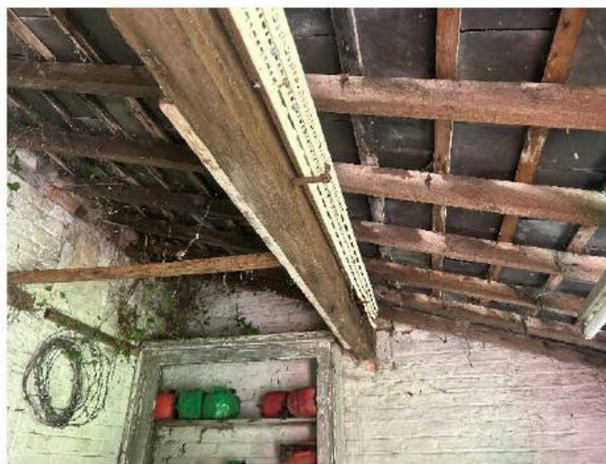
Plate 5 - View of roof within Building 5.
