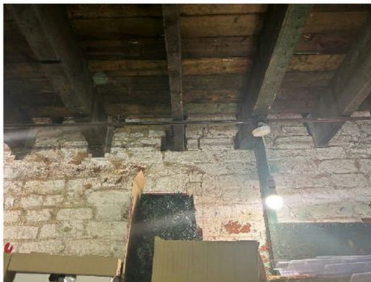
Plate 4 - Loft void within western section of Building 2.
