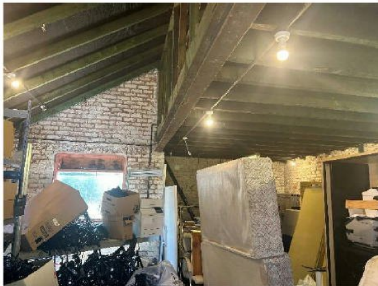
Plate 3 - Loft void within western section of Building 2.
