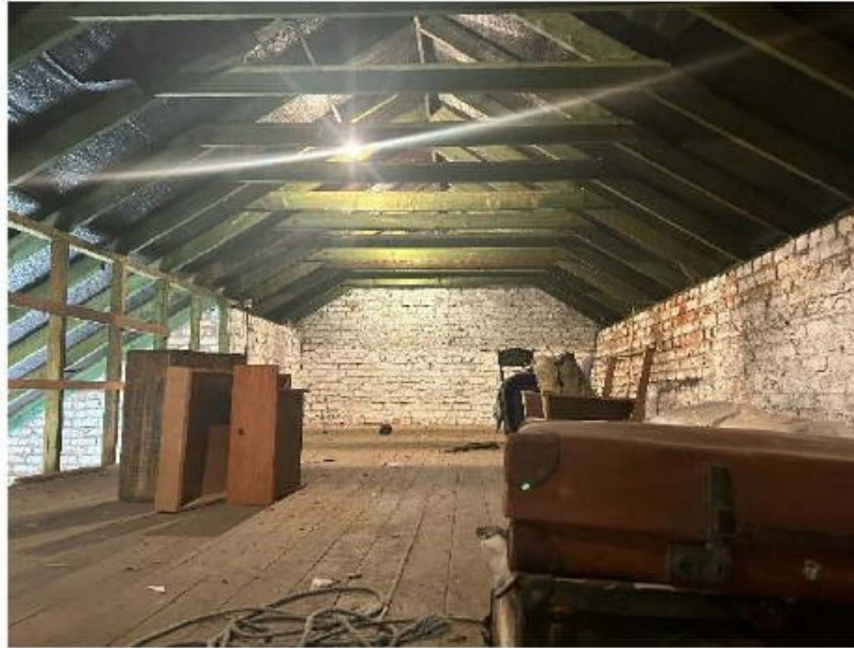
Plate 2 - Loft void within western section of Building 2.
