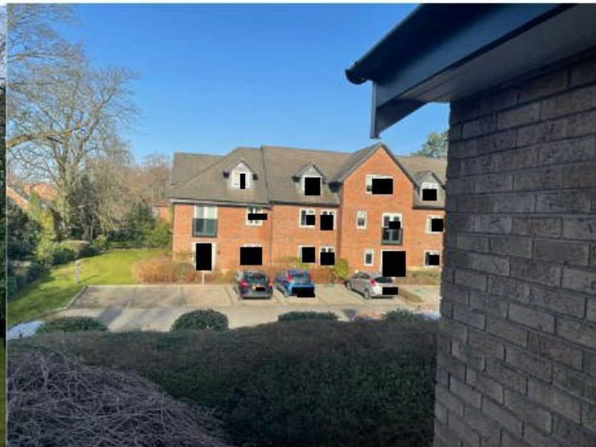
View from 41 Ashlands showing existing Michael Court building. Lower profile and Juliet balconies
