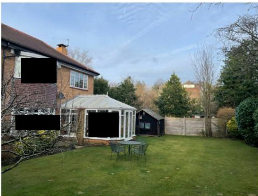
View of rear of 41 Ashlands with 2 storey bay showing again the clear view into the site
