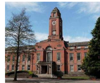
TRAFFORD TOWN HALL - GRADE 2 LISTED
