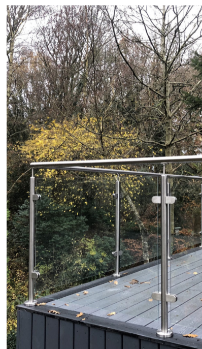
4 1100mm Glass balustrades on balconies
