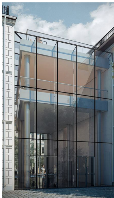
1 Curtain walling to the ground floor commercial units
