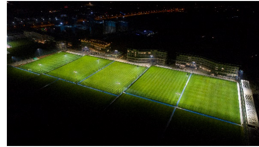
2019/20 – Dalian Wanda Training Facility, Dalian, China Concept, detailed design and installation monitoring for a new elite level training facility in Dalian China Client: Wanda
