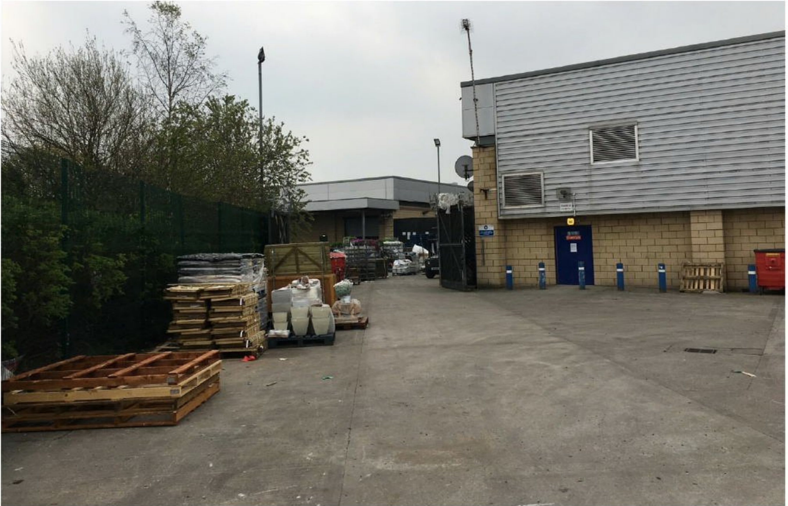
Service yard to north of Homebase building.
