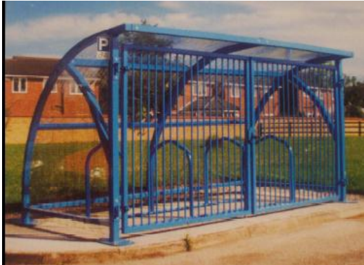
Fig 8: freestanding, covered, secure compound containing Sheffield stands
