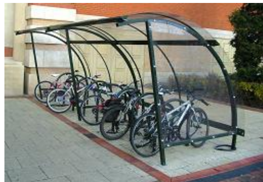
Fig 7: long stay open access cycle parking using covered Sheffield stands
