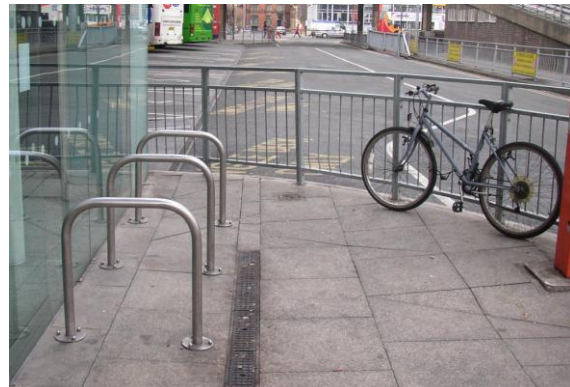
Fig 5: Sheffield stands allow a bicycle to be rested against a steel frame and the A-frame of the bicycle to be secured. This example is placed with sufficient clearances to allow correct use.
