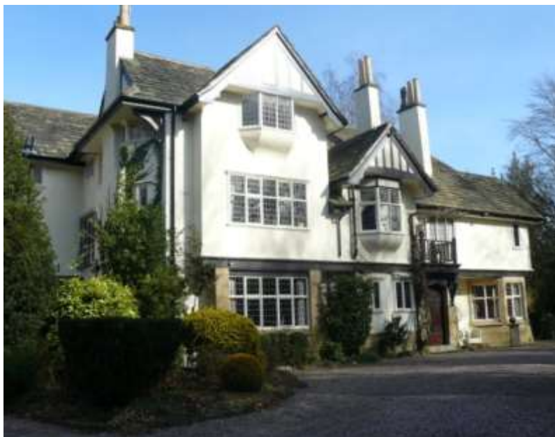
An example of the characteristic varied roofline, use of half-timbering and render
