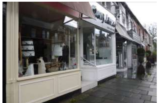
Original shop fronts with stall risers, slender glazing bars and panelling. The fascias are not appropriate
