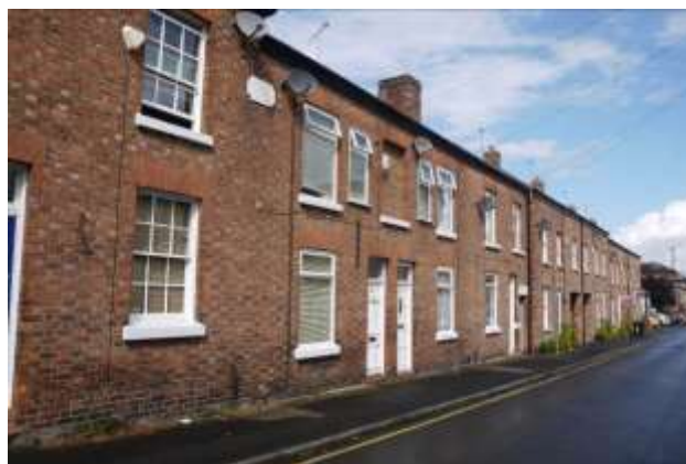
Simple terraces on New Street harmed by inappropriate style doors, uPVC windows and intrusive satellite dishes
