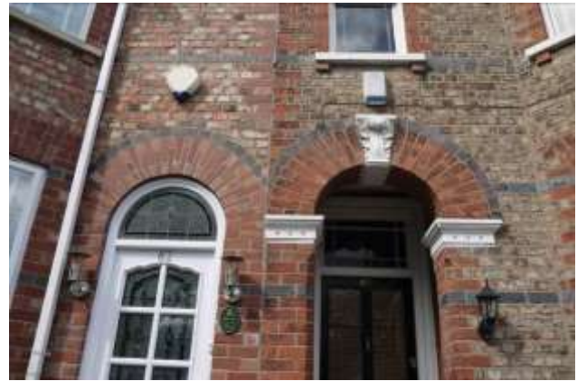
Additions to the ends of terraces attempt to emulate the existing structures but fall short on detailing such as decorative key stones and corbels
