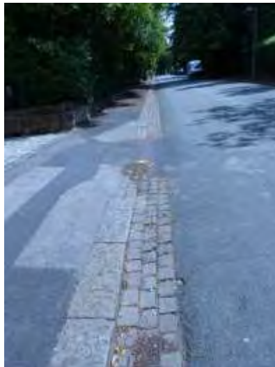
An example of cobbled setts, historic kerbstones and ad hoc tarmac repairs, as well as a good example of modern setts to the driveway.
