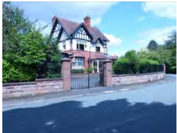
Replacement gate posts on Howard Drive, which are too tall and of an incongruous design. The capping along the original wall is also inappropriate
