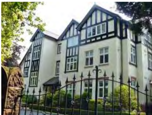
A modern apartment building on Harrop Road, which is identified in the Appraisal as detracting for its design and scale which does not befit the semi-rural character of the Conservation Area
