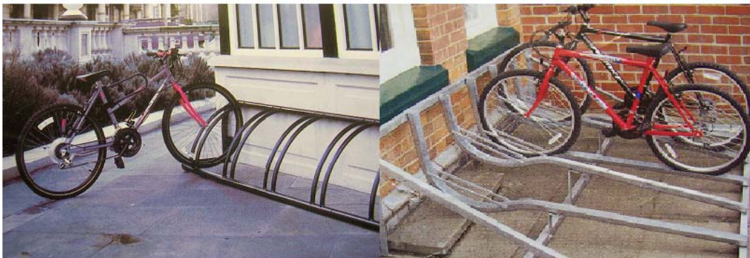
Fig 4 Unsuitable racks that only allow the front or back wheel to be secured.
