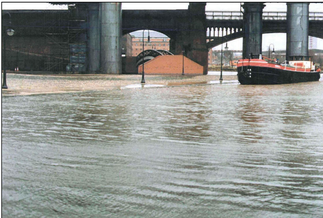
Figure 2-4: Bridgewater Canal during December 1991 Flooding
