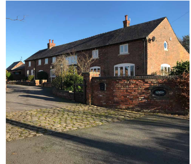
Figure 35: Brick, terraced houses at Higher Carr Green Farm
