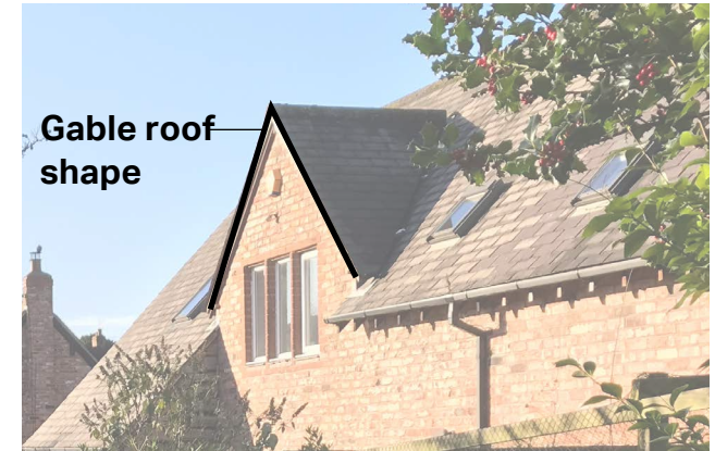
Figure 49: Gable roofed wall dormer and skylights
