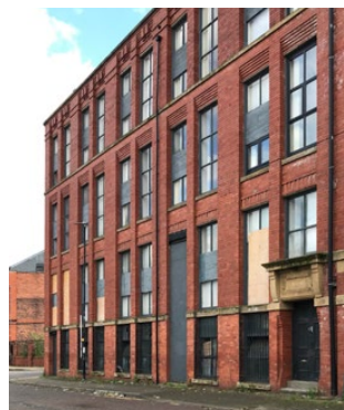
Openings such as doors and windows are expressed using devices like corbel detailing and material changes.
