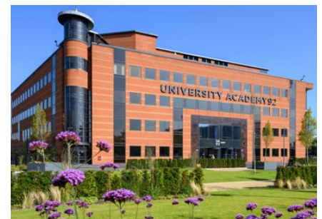
Former Kellogg's building
