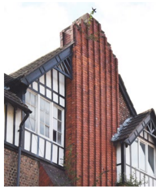
Ribbed brickwork, decorative metalwork and corbel details can be observed on buildings in the local area.
