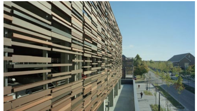
Garland Centre, Multi storey car park
