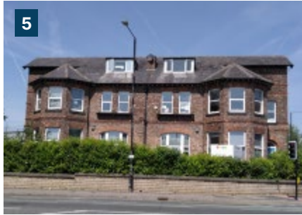
Victorian villas to Talbot Road
