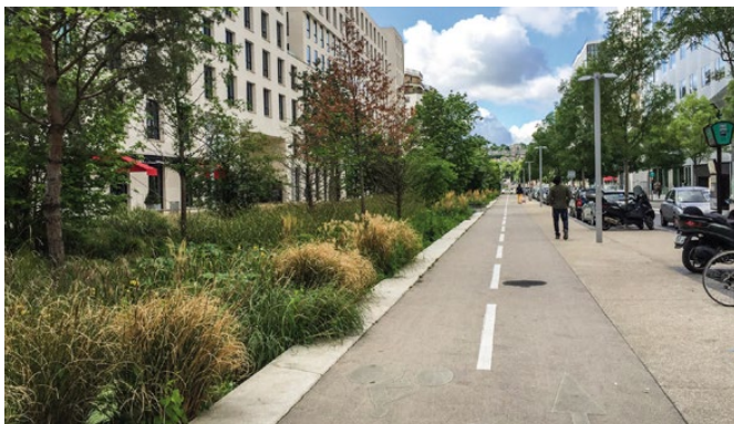
SUDS as street feature - Parc de Billancourt, Paris
