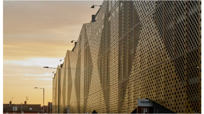
Crown car park, façade
