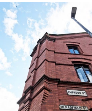
Turning the corner with the use of a chamfer appears on several buildings such as Vryniew House on Talbot Road, Trafford Town Hall and within the Empress Conservation Area.
