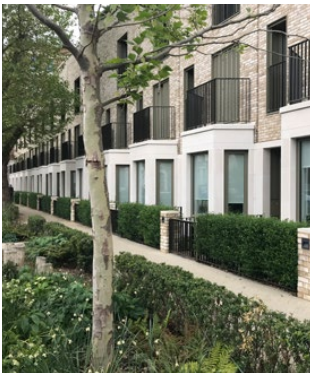
Canted, bow and oriel bay windows are all found in the local area.
