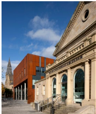
Broadcasting Place, Leeds
