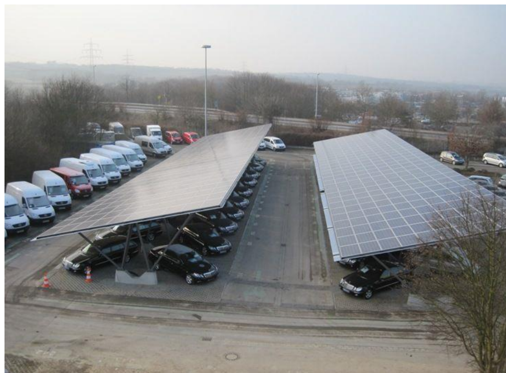
Figure 4-4 - Example of a solar carport, giving the land a double use
