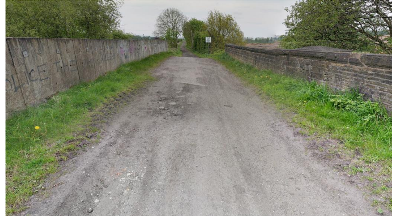
Figure 2-15 - Existing bridge over Carrington Greenway
