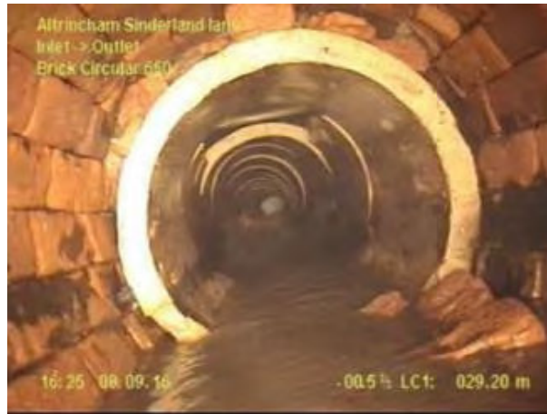
Figure 33 - View inside the culvert from cctv survey
