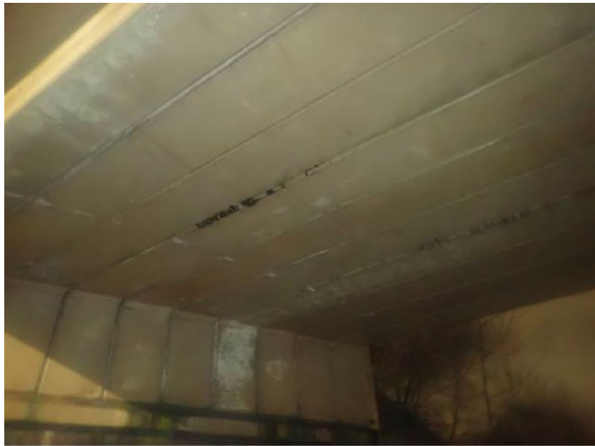
Figure 19 - View under the bridge deck
