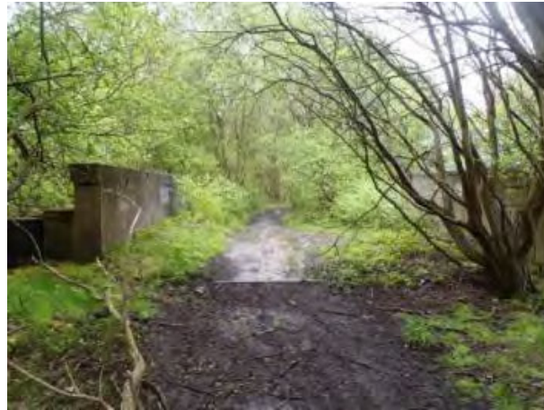
Figure 30 - View over the structure
