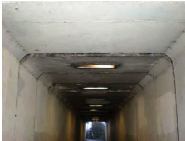
Figure 16 - View inside of the structure
