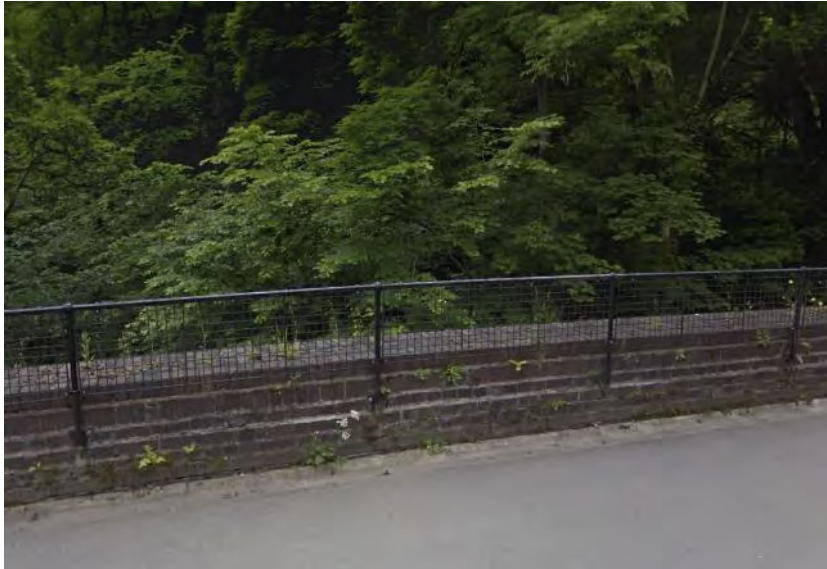
Figure 62 – Parapet extension example for masonry (Monsal Trail)
