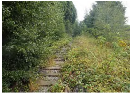
Figure 43 - View over the structure
