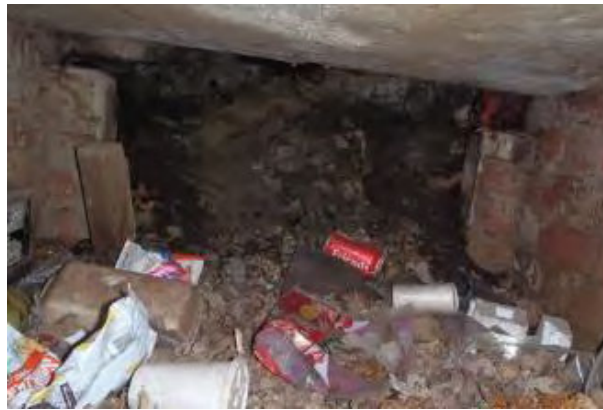
Figure 38 - View insider the structure
