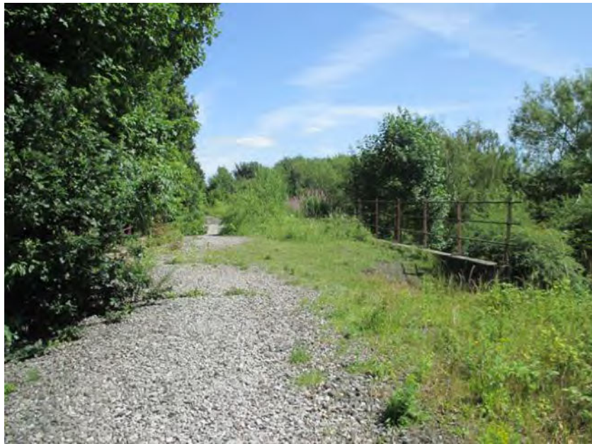
Figure 46 - View over the structure
