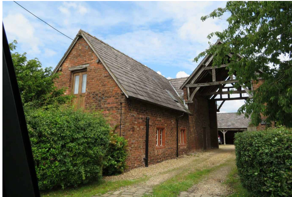
Figure 06: Barn to south east of Birch Farmhouse
