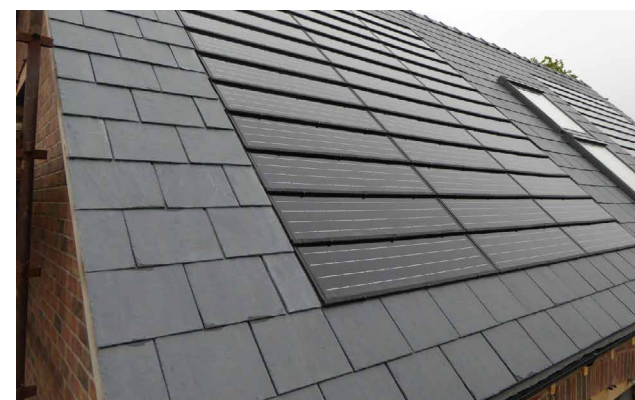
Figure 53: Solar slate example image
