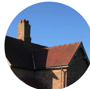
Figure 63: Clay roof tiles
