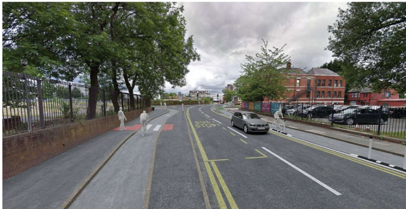
Figure 2: Talbot Road looking Eastbound.
