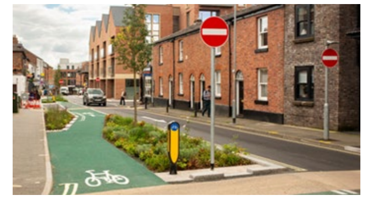
Before & After Regent Road: now a one way from the junction of Railway Street and Market Street. A new segregated contraflow cycle lane which is lined with ‘rain gardens’ that introduce trees, green infrastructure and SuDS to the area.
