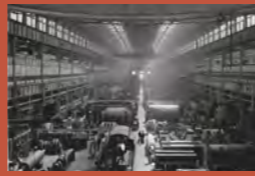
Associated Electrical Industries Ltd. in the 1930s
