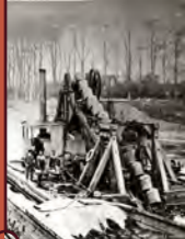
Construction of the Manchester Ship Canal
