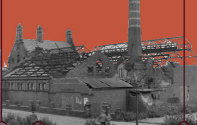
Bomb damage in the 1940s
