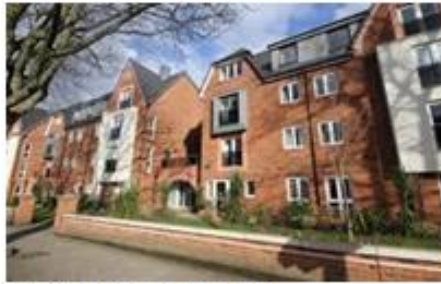
Oakfield Court, Urmston
