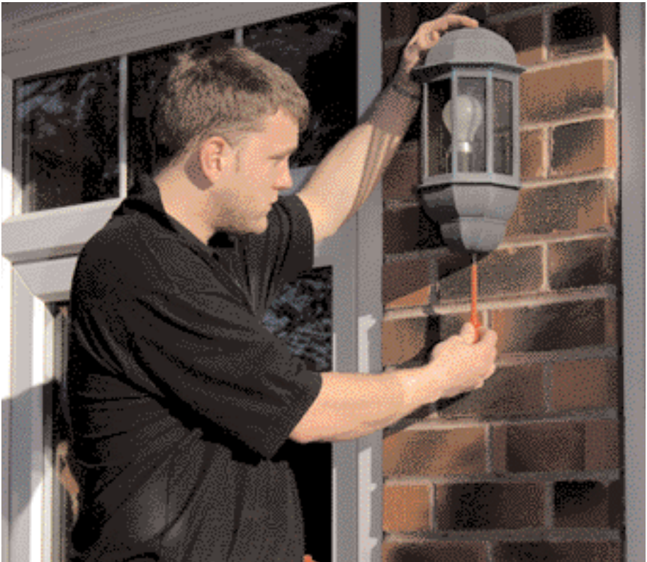
Outside Lighting subject to Part P
