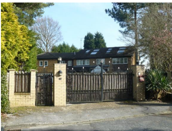
Photograph 19: Brick Piers with Metal Gates, Blenheim Road
