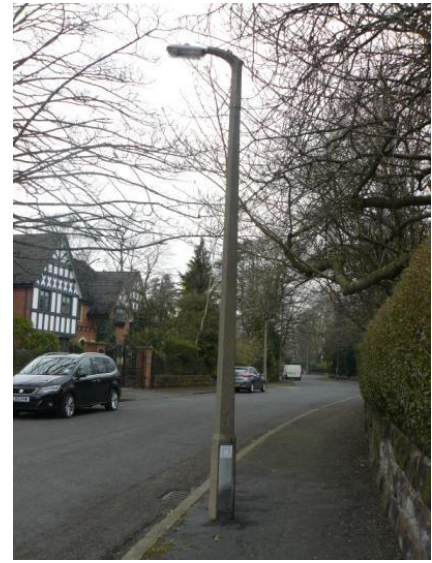
Photograph 30: Concrete Lamp Post
