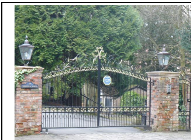
Photograph 27: Modern Gates and Gate Piers
