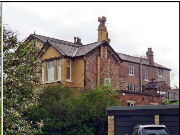
Photograph 104: Rear Elevation of Byefield and Lynwood
