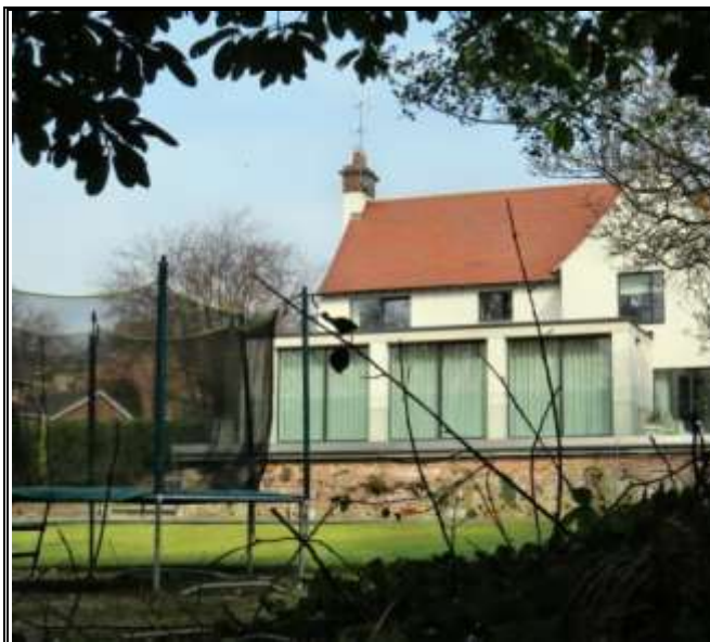
Photograph 149: Modern Extension to Rear, Talbot Road:
