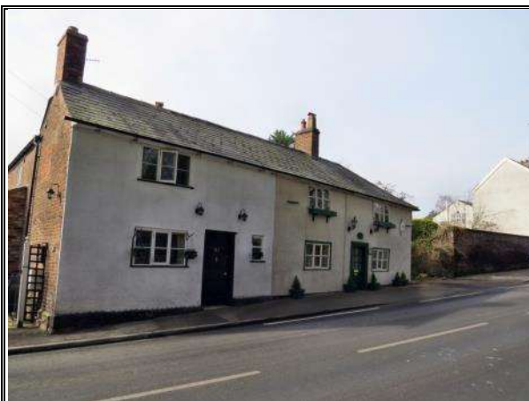
Photograph 33 :Crossvale Cottage, 83-85 Langham Road
