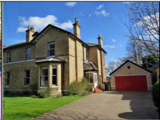
Photograph 146: Intrusive Colour of Garage Door
