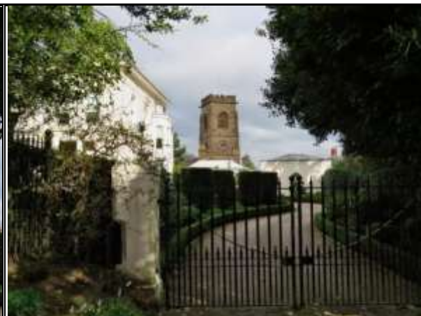
Photograph 106: Kirklee with View of St Mary's and New Garage in Foreground.
