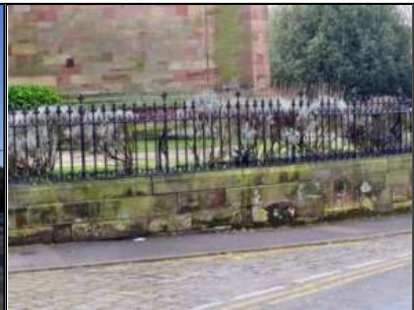
Photograph 8: Listed Railing and Wall, St Mary's Church
