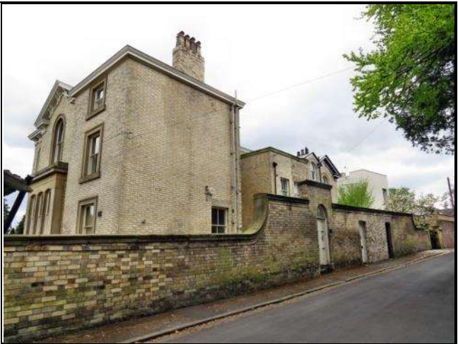
Photograph 148 Extension and Loss of Architectural Detail, 22 East Downs Road
