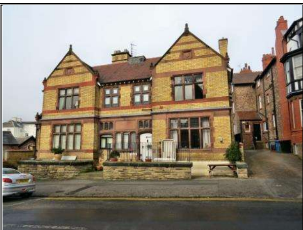
Photograph 34: Church Brow Flats
