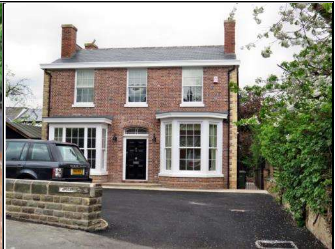
Photograph 138: Infill Building with no Soft Landscaping (Applegate House, West Road)
