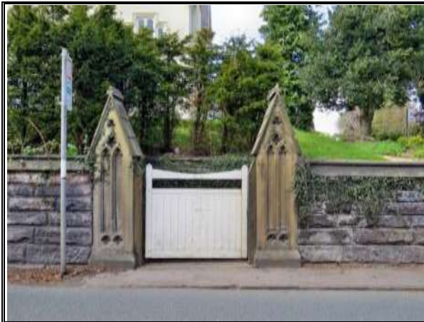
Photograph 83: Pedestrian Gate and Posts, 16 Langham Road
