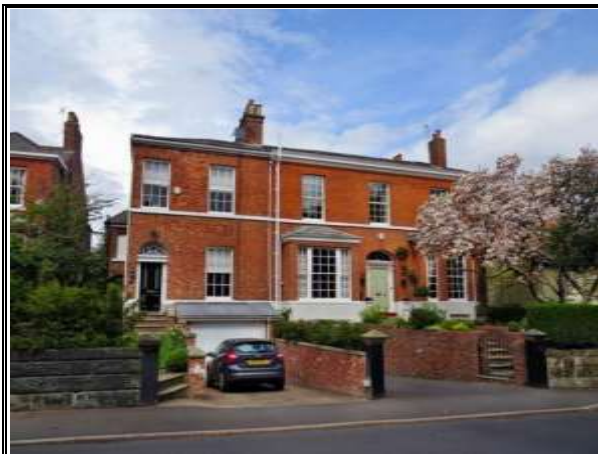
Photograph 87: Altered Boundary and Garage Inserted to Basement, Stamford Road
