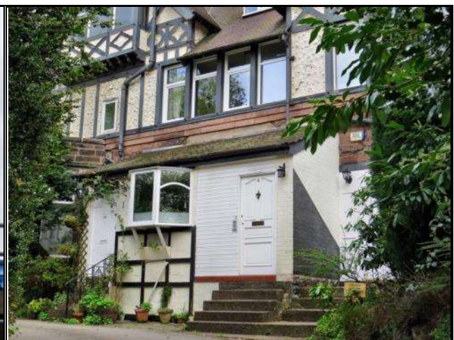
Photograph 136: 72 Stamford Road Converted to Flats
