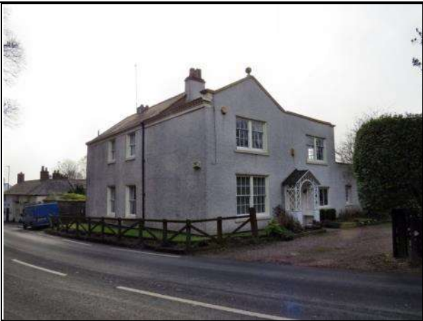
Photograph 32: Vale House, Langham Road
