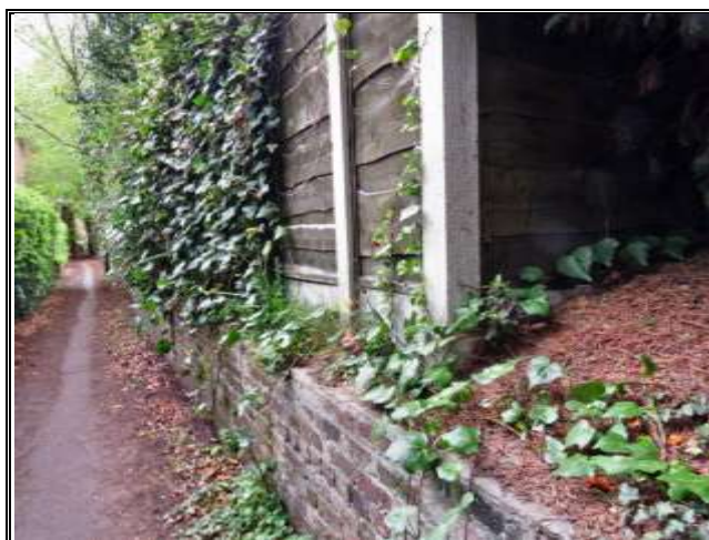
Photograph 153: Fencing on The Narrows
