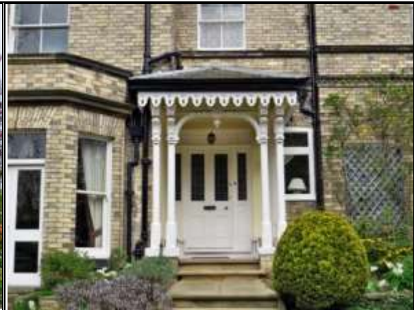
Photograph 100: Detail of High Row
