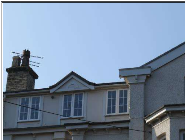
Photograph 139: Roof Extension, The Firs
