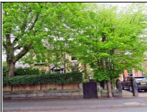
Photograph 21: Boundary Wall, Fence, Stone Gateposts (11 Stamford Road)
