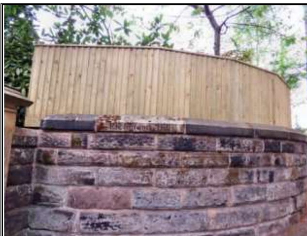
Photograph 161: New Fence, Richmond Hill
