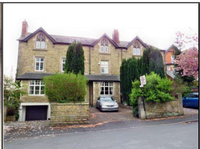
Photograph 144: Garage in Basement, West Road
