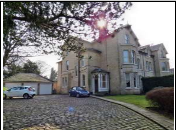
Photograph 12: Westholme, with Porch
