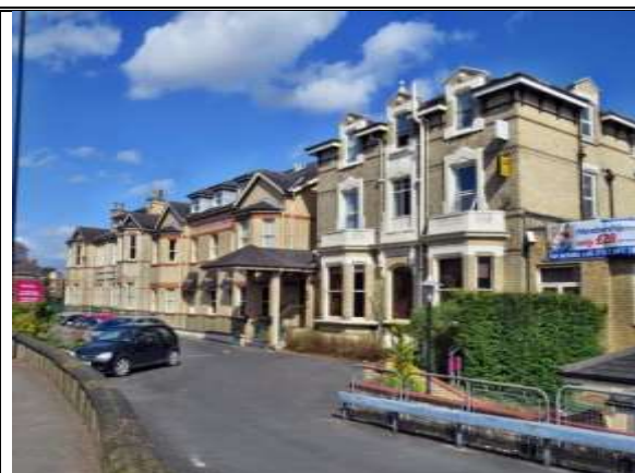
Photograph 78: The former Bowdon Hydro
