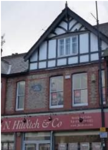
Typical shop buildings along Ashley Road
