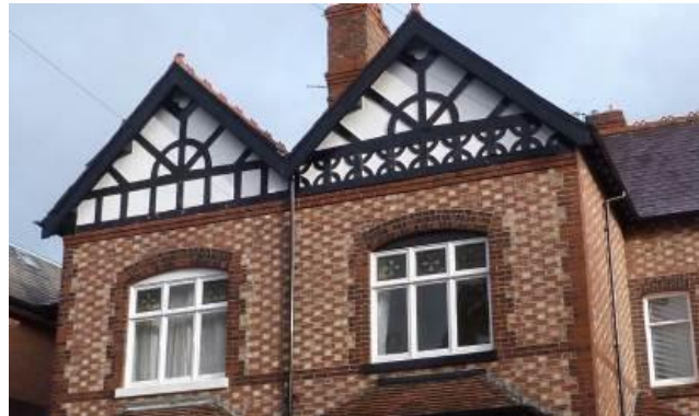
Flemish bond brickwork and timber-framing
