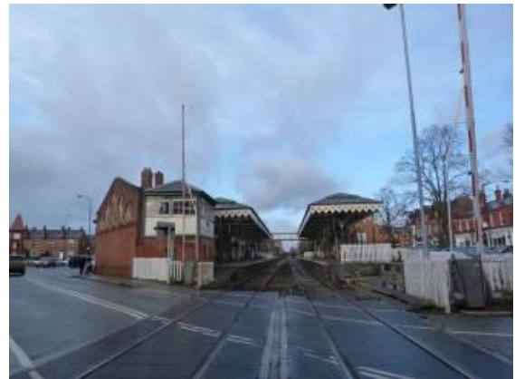
View north along the railway lines past the listed station buildings
