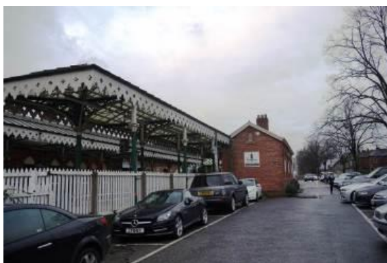
View of the car park to the east of the station
