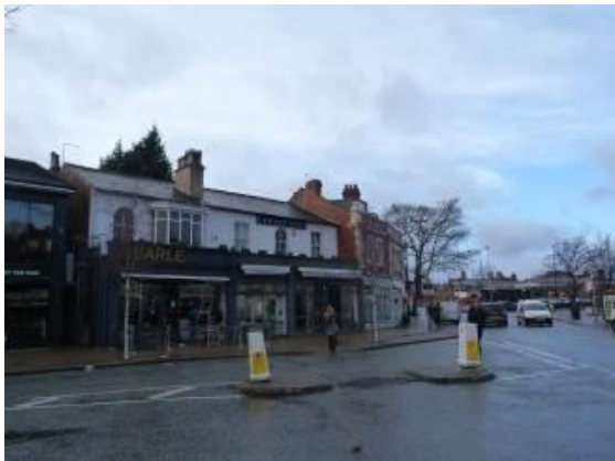
View looking west along Ashley Road towards the station
