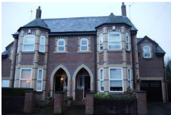
Modern replacements on Spring Road
