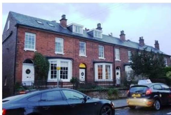
Example of the terracing along Ashley Road
