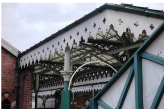
Detail of the east platform canopy
