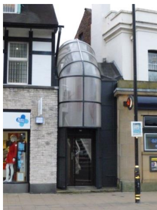
Intrusive glazed in-fill between 197 and 197b Ashley Road
