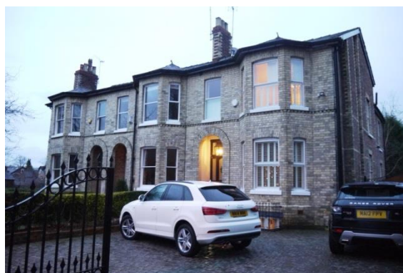
Annex extension to No. 78 Ashley Road
