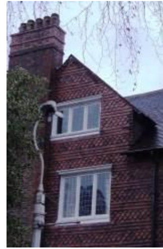
Arts and Crafts details such as chimney stacks, tile-hanging and leaded glazing
