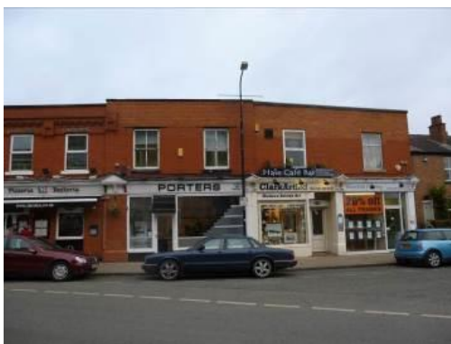
Ornamented parapet replaced to retail units on Hale View
