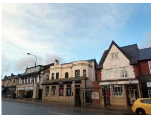
Eclectic architecture and shop fronts on Ashley Road
