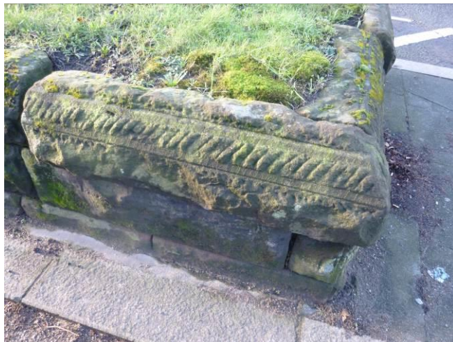
Retaining wall to Manchester Road central island
