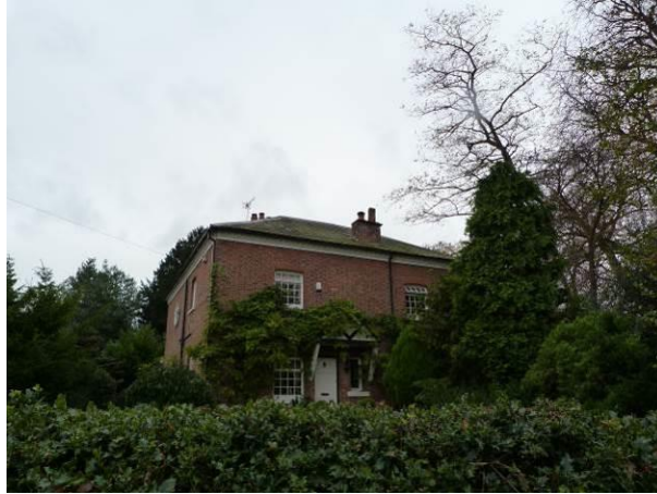
The Lodge to the former Oldfield Hall
