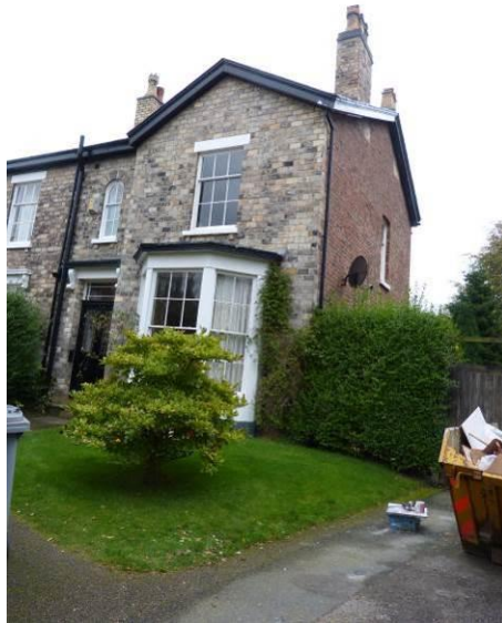
No. 16 Sandiway Place
