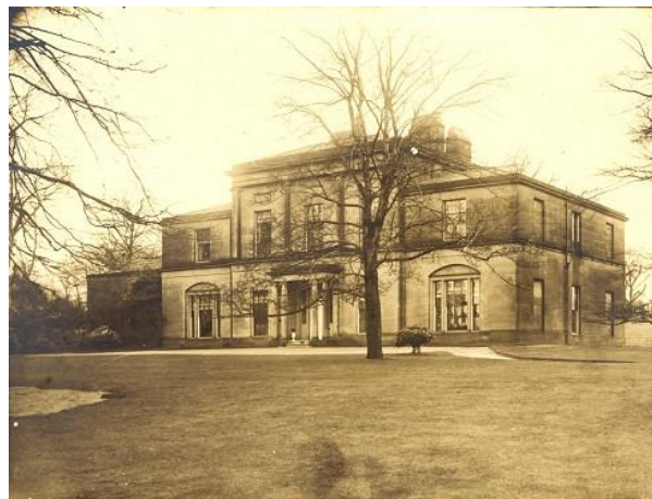
The (much-altered) house prior to its demolition in 1916 (TL4516, Trafford Lifetimes)
