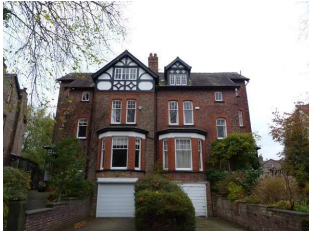
Nos. 25 and 27 Burlington Road
