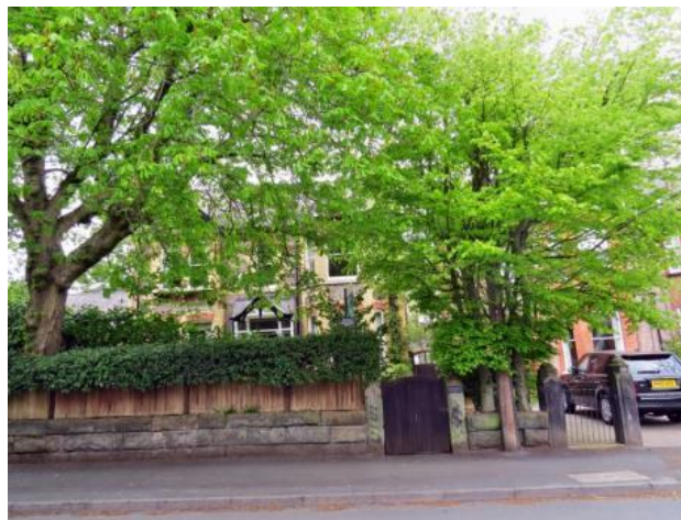
Boundary treatment, Stamford Road. Note the historic low stone wall and gate posts, but incongruous gate, which is too big, and inappropriate use of timber fencing
