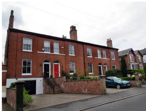
30-36 Stamford Road - a balanced classical terrace but with a harmful basement extension and front drive
