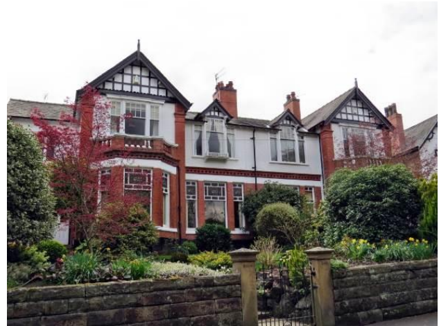
surviving historic windows, Stamford Road
