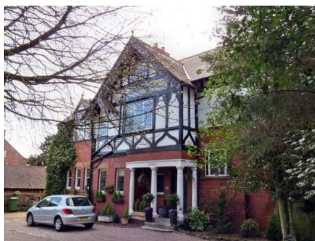
The Red House, Langham Road - combining Arts & Crafts with Cheshire Revival features
