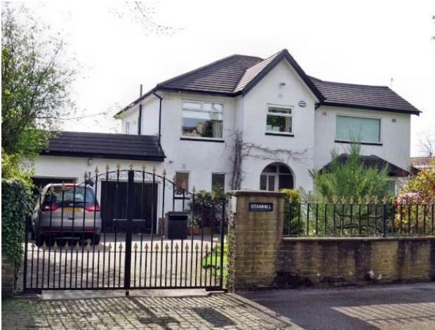
Inappropriate replacement windows on Delamar Road
