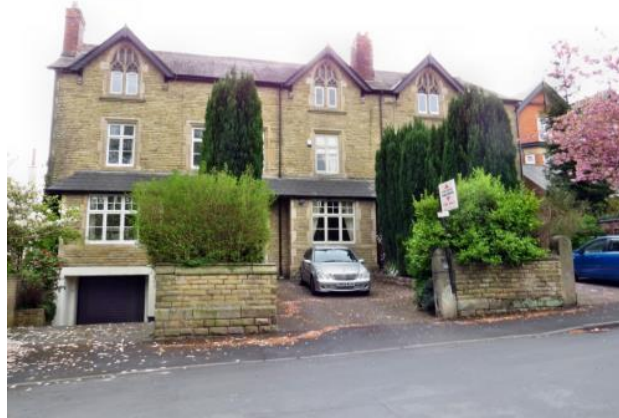
Substantial re-landscaping for the provision of a basement garage which has resulted in the elongation and mis-balance of the main elevation, West Road
