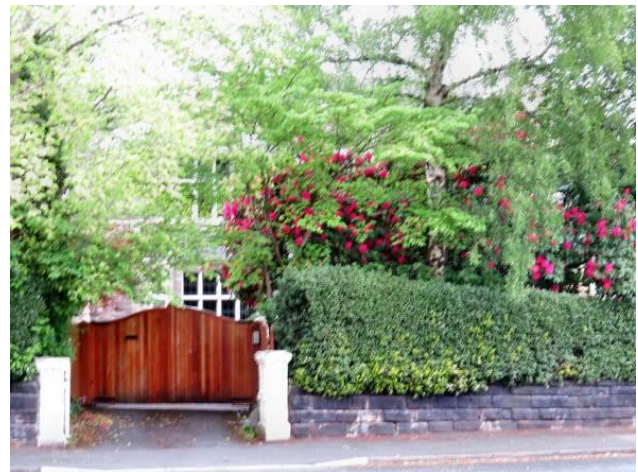
Obtrusive gates which do not respect the proportions of the gate posts, Heald Road
