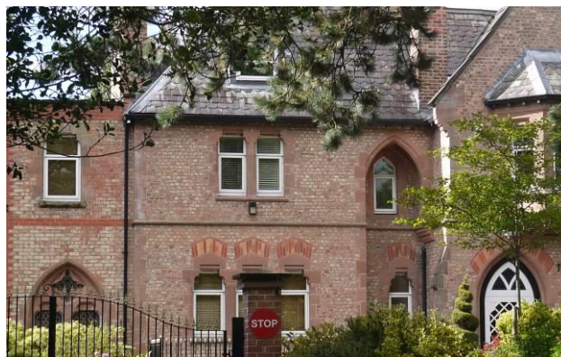
Gothic architecture with plate tracery and arched openings. Note the decorative slates and a high quality use of the local brown bricks.
