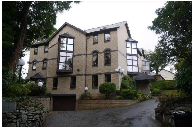
Beaupré, Bowdon Road, intrusive 20th century development on an historic plot. The use of reflective glazing is particularly inappropriate.
