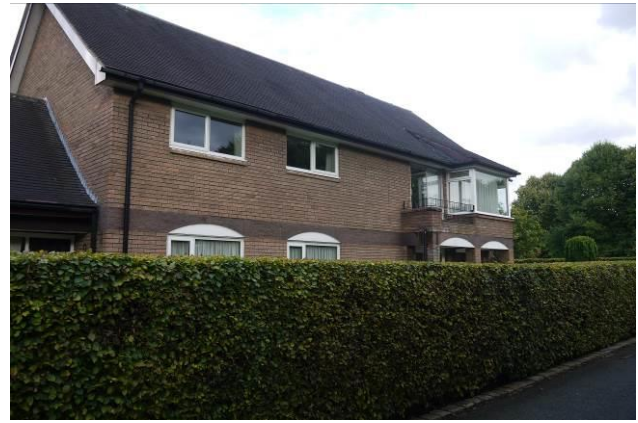
Example of the 1970s cul-de-sac housing within Green Courts
