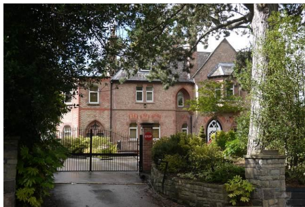
Typical materials include local brown brick, decorative Welsh slate, timber windows and stone details, Morningside, Highgate Road
