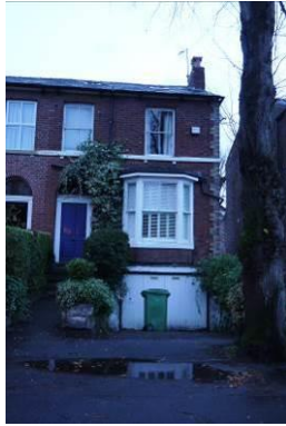
Inappropriate converted basement garage at 12 Spring Road
