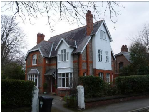
Arts & Crafts architecture on Lisson Grove incorporating polychromatic brickwork, rendering, half-timbering, timber porches and tall chimneys
