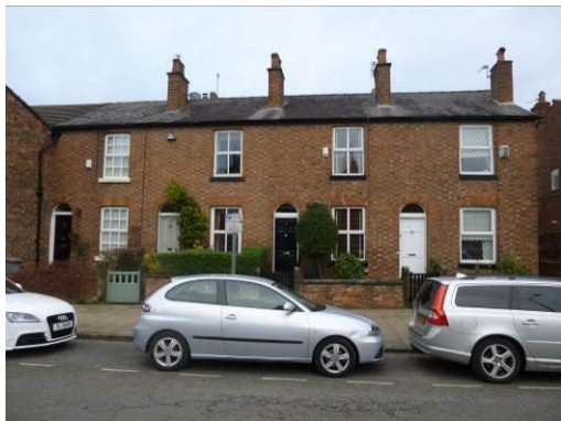
Simple early 19 th century façades with replacement doors and uPVC windows. Leaded glazing is inappropriate
