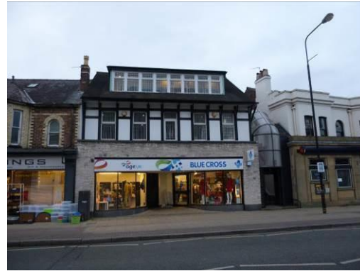
Inappropriate stone cladding on the ground floor and signage that does not respect the historic character of the Conservation Area
