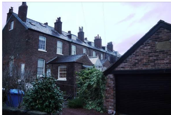
Rear elevations along the residential dwellings of Ashley Road, within Character Zone D
