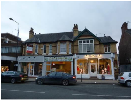
Traditional shop front at 186 Ashley Road (right), next to two inappropriate modern shop fronts (190-188 Ashley Road) with large fascias and aluminium framed glazing
