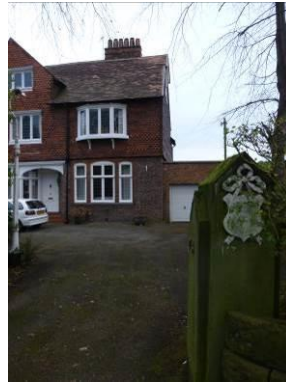
Original stone gate pier at 103 Ashley Road
