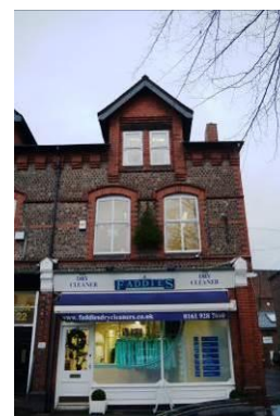
Detail of the late Victorian brickwork including header bond, red brick window surrounds and brick dentilled eaves. The shop front is also original.
