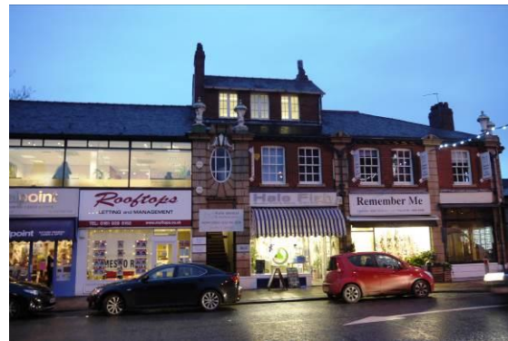
Inappropriate infill development (left) at 161 Ashley Road
