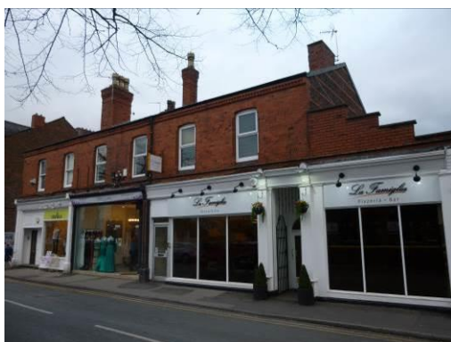
Inappropriate shop front with no stall riser and a large expanse of glass with no glazing bars at 16 Victoria Road (Dress 2 Party). The darkened glazing at 12-14 is also not appropriate.
