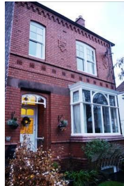
Decorative terracotta and original ground floor windows in this house of 1899
