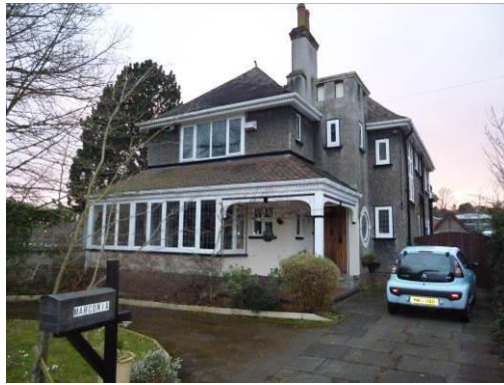
Note the original leaded windows on the ground floor and the original external pebbledash
