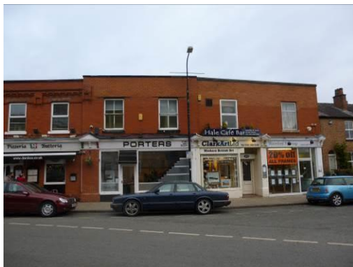
Traditional shop front features such as capitals, pilasters and recessed doorways in Character Zone A. Window signage is inappropriate.
