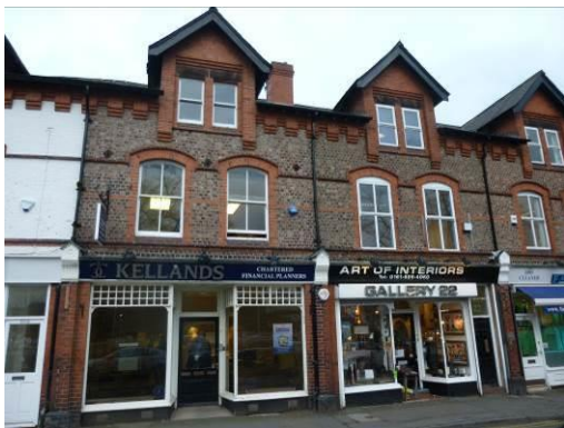
Historic shop fronts along Victoria Road with slim timber glazing bars and recessed doorways (Character Zone A). The glazing bars to the right were removed in 2015, which is harmful to significance.
