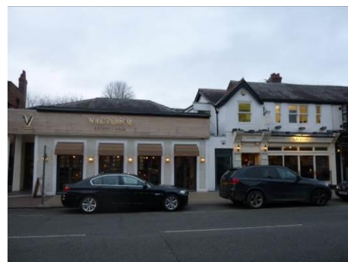
Intrusive stone and timber cladding on an historic building at 169 Ashley Road
