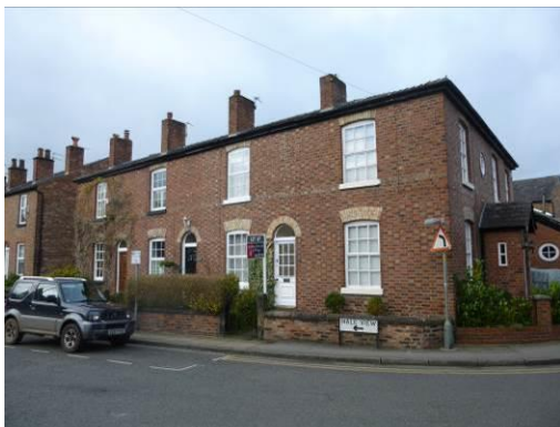
Early 19th century architecture including burnt header bricks, sash windows and simple façades
