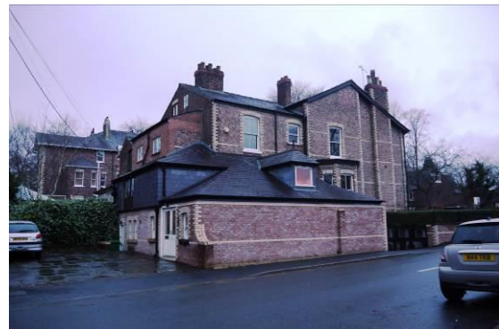
Inappropriate modern annex at no. 78 Ashley Road
