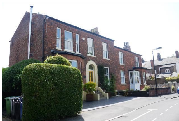
Edale House and Rose Lea showing good quality buildings with some inappropriate alterations and loss of boundary walls.
