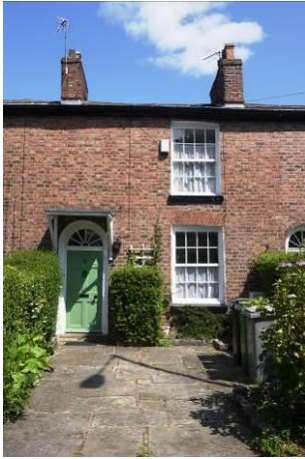
Example of the cottages on Sandiway Road. Note the inappropriate asphalt-covered porch and the loss of the front garden.
