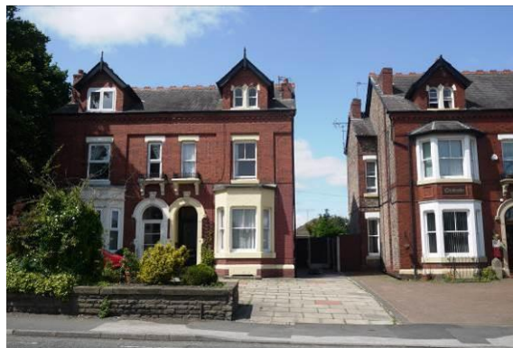
The two larger Edwardian houses on the Manchester Road. Some boundary treatments have been lost to create driveways.
