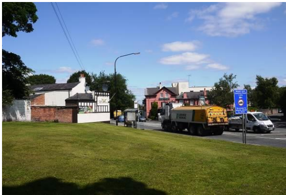
Intrusive signage and busy traffic along the A56, cutting through the Conservation Area
