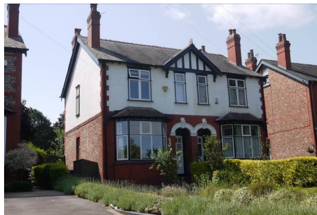
The palette of materials used across the Conservation Area include slate roofs and red brick, half-timbering, stained glass and leaded-lights, timber windows, clay chimney pots. Pebble-dash can be found along Oldfield Road but is not common.
