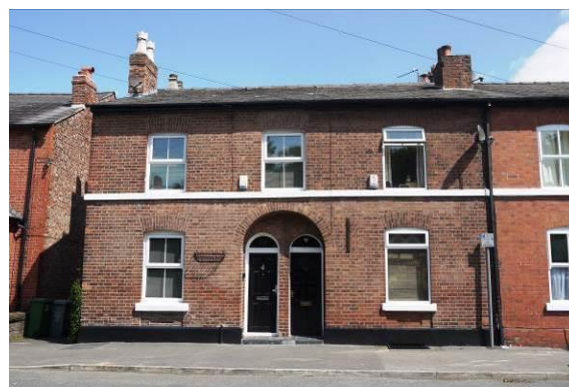
Example of the late Georgian style houses on the north side of Oldfield Road, nos. 20-26
