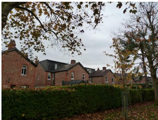
The rear of properties on the north side of Oldfield Road
