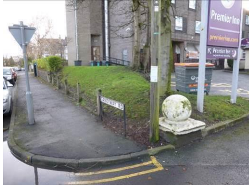
An eclectic mix of signage, poor public realm and intrusive additions to the buildings create a cluttered and unsightly streetscape
