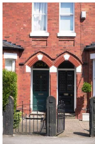
Original doors along Oldfield Road at nos. 48-58
