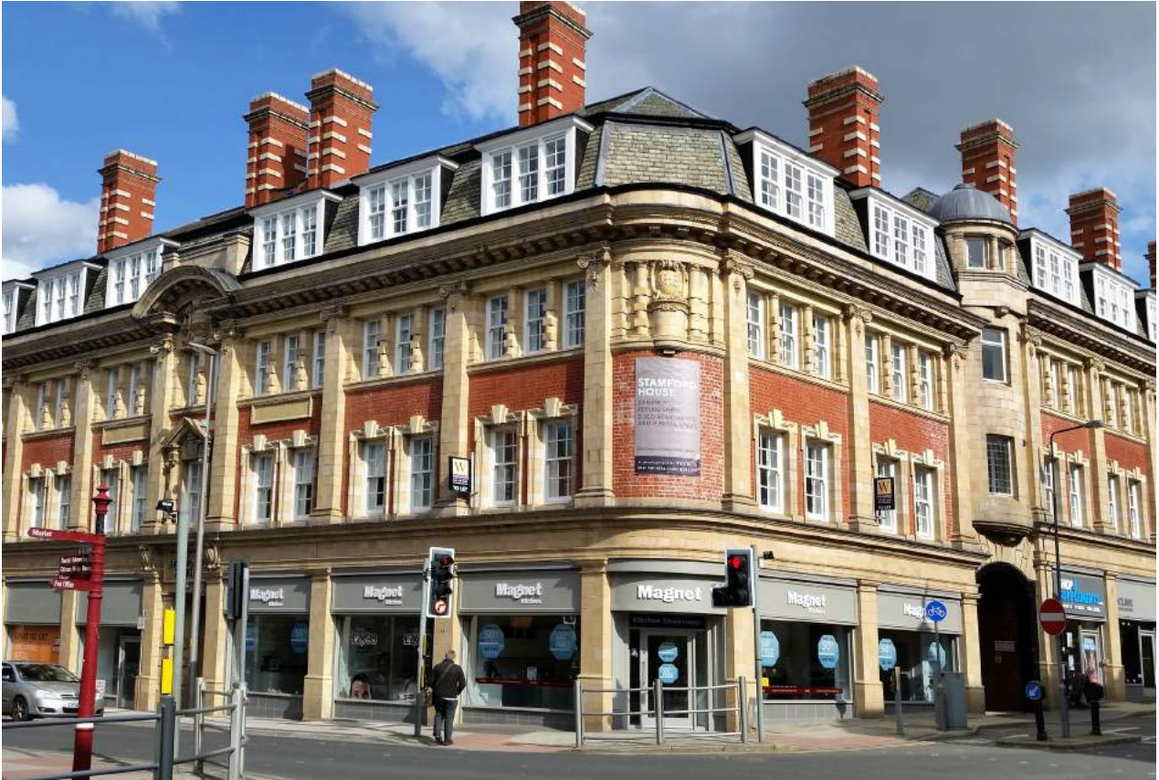
Station buildings at the corner of Stamford New Road and Moss Lane, carefully restored externally, with the traditional shop front design reinstated, during the conversion of the upper office floors for residential use.
