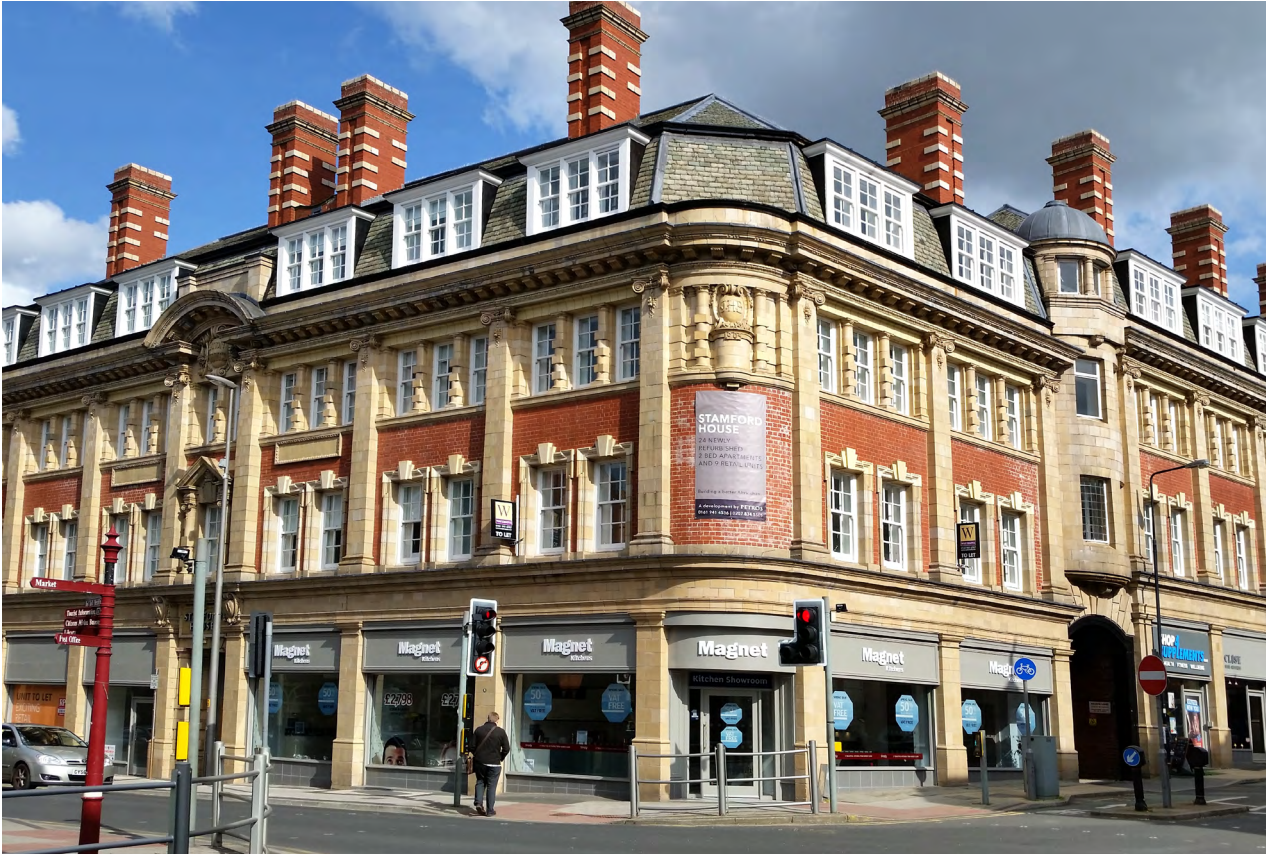
Station buildings at the corner of Stamford New Road and Moss Lane, carefully restored externally, with the traditional shop front design reinstated, during the conversion of the upper office floors for residential use.
