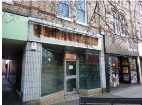
Photograph 13: Vacant shop/deteriorating signage
