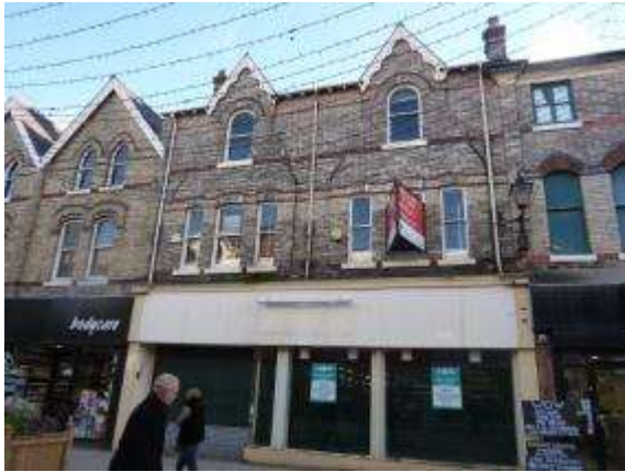
Photograph 12: Vacant shop with intrusive 'to let' board.
