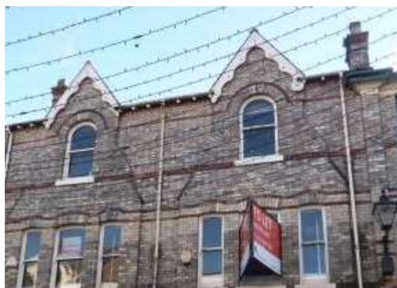
Photograph 17: Decorative barge boards
