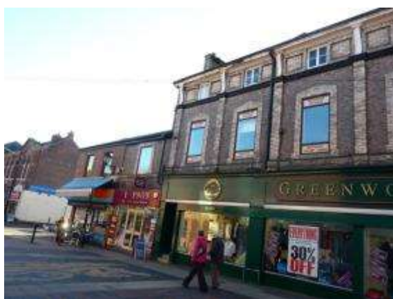
Photograph 6: 69 George Street, an example of classical revival with polychromatic brick pilasters and façade divided into classical proportions
