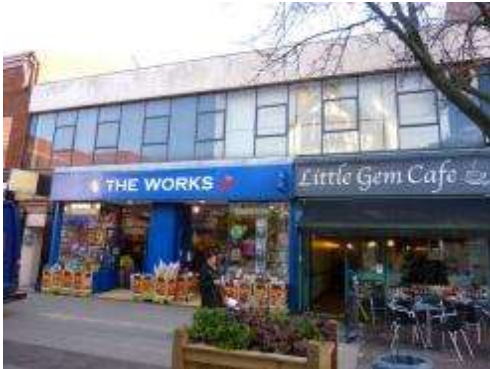
Photograph 8: Inappropriate signage & shop front, No. 77 George Street
