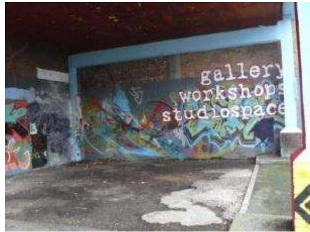
Photograph 25: Space underneath the intrusive structure to rear of 72 George Street
