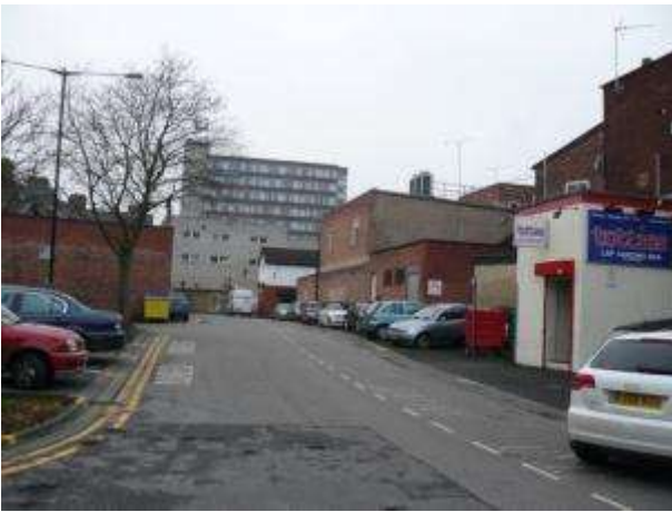
Photograph 24: Extensions facing onto The Causeway
