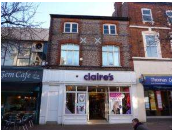
Photograph 10: No. 83 George Street; appropriatereplacement shop front with exception of the signage which is considered intrusive
