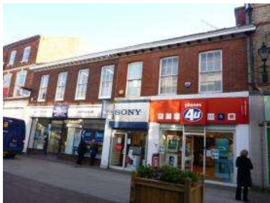
Photograph 4: Classically styled properties evident from the upper storeys
