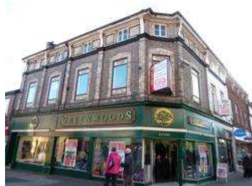
Photograph 9: Appropriate shop front design, No. 69 George Street
