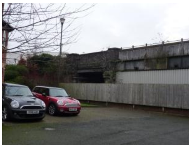
Photograph 31: Former railway bridge
