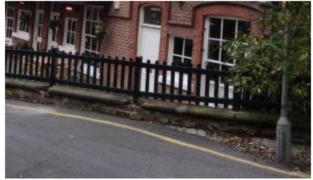
Photograph 43: Wall outside No. 13
