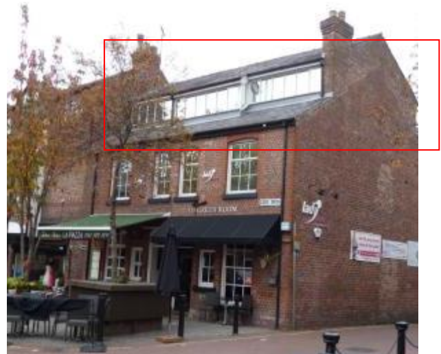
Photograph 25: 20th century extension to roofscape
