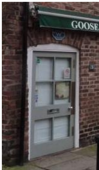
Photograph 18: Door with soldier arch
