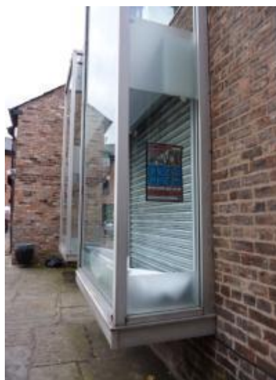
Photograph 6: 20th century windows with internal metal shutters
