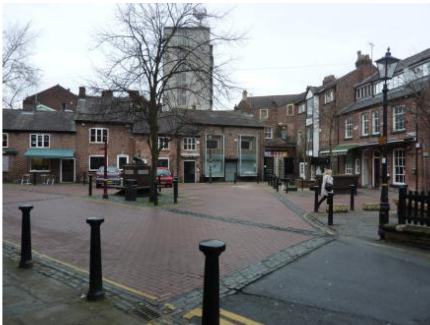
Photograph 37: View looking northwest from the former railway bridge
