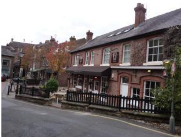
Photograph 30: Brick wall with stone coping
