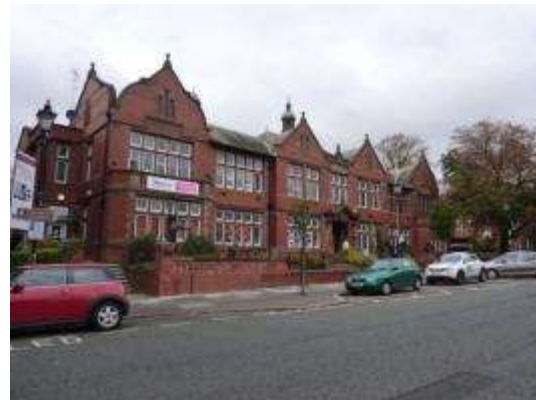
Photograph 42: Altrincham Town Hall, Market Street
