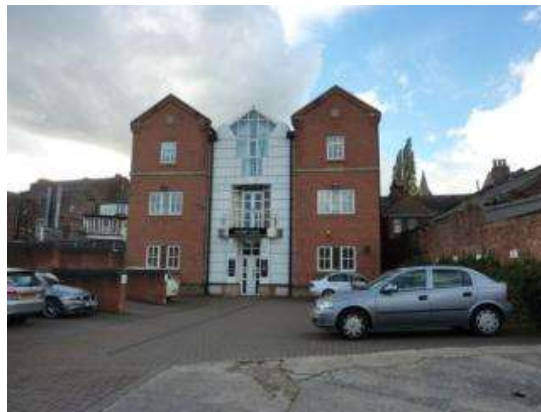
Photograph 99: 20th century extensions to properties fronting Church Street t
