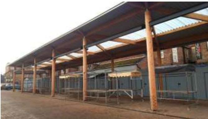
Photograph 57: Refurbished Lower Market, Central Way
