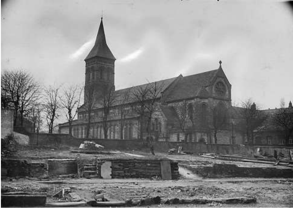
Photograph 5: Demolition on Church Street, 1938 (Trafford Lifetimes, TL3695)
