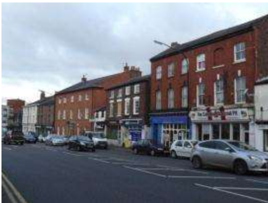
Photograph 26: Commercial properties on Church Street
