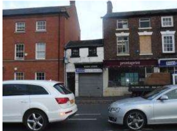
Photograph 31: 18 Church Street displaying external roller shutter and inappropriate signage at Prontoprint
