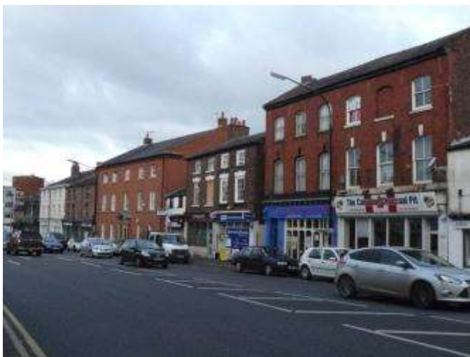
Photograph 24: Commercial Properties on Market Street
