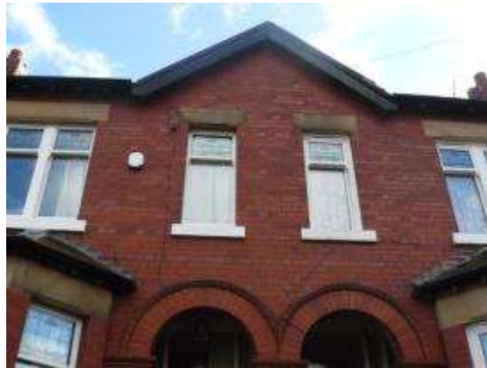
Photograph 77: Timber sash windows with decorative glass
