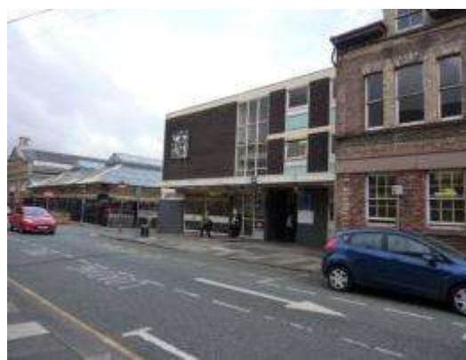
Photograph 35: Mid 20th-21st century extension to Altrincham General Hospital
