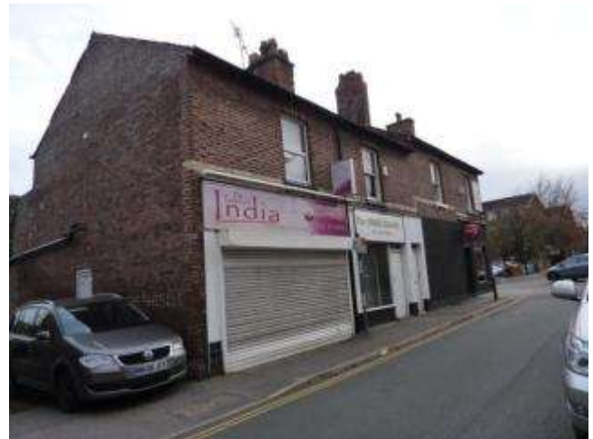
Photograph 89: Intrusive signage and roller shutters
