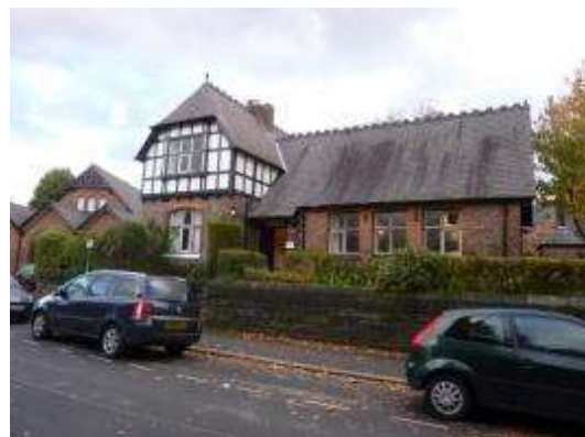
Photograph 69: Former school building, Sylvan Grove
