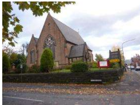
Photograph 71: The Unitarian Chapel, Dunham Rd
