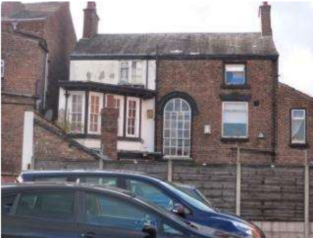
Photograph 85: Rear of properties on Church Street
