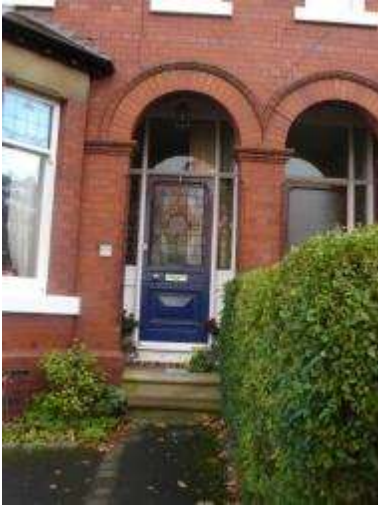
Photograph 76: Semi-circular doorway with decorative glazed door
