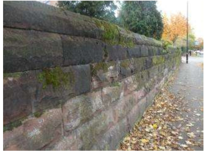
Photograph 14: Sandstonewall fronting Church Street
