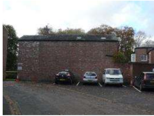
Photograph 75: Townfield house estate buildings
