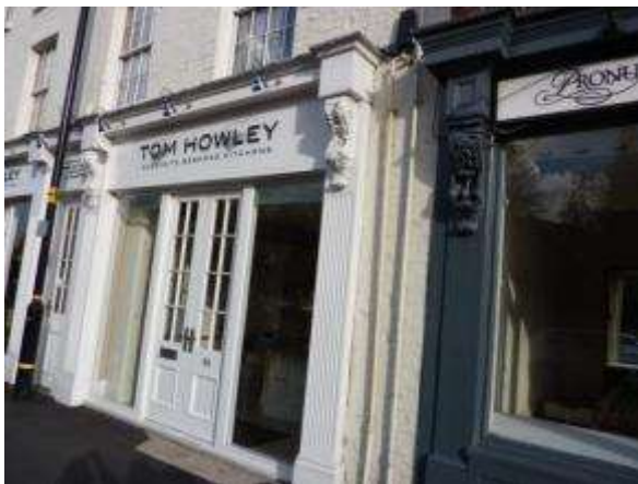
Photograph 28: Traditional painted timber shop fronts with decorative pilasters, consoles, minimal fascias and signage with external spot lighting
