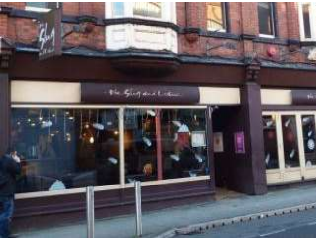
Photograph 19: Shop front with timber riser and corbels
