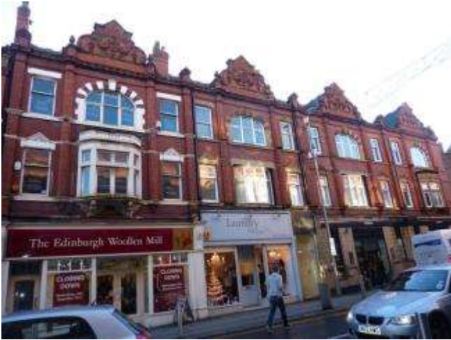
Photograph 10: 15-21 Stamford New Road
