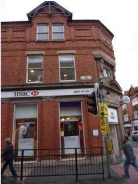
Photograph 17: No. 13 Stamford New Road
