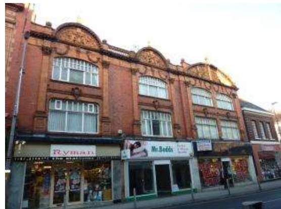
Photograph 28 : Prominent gables to front façade
