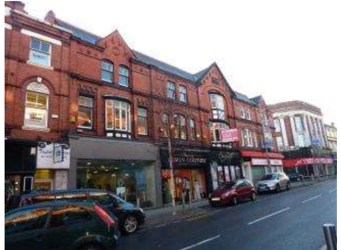
Photograph 7 : Three storey brick terrace with slate roof
