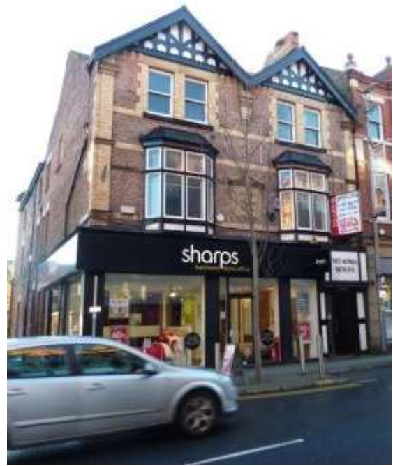
Photograph 22: 21st century intrusive shop front
