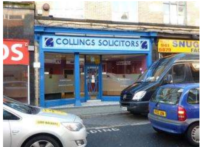
Photograph 20: Shop front with remaining cornice and corbels
