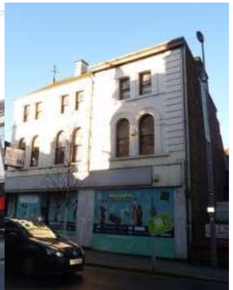
Photograph 14: 48-50 Stamford New Road
