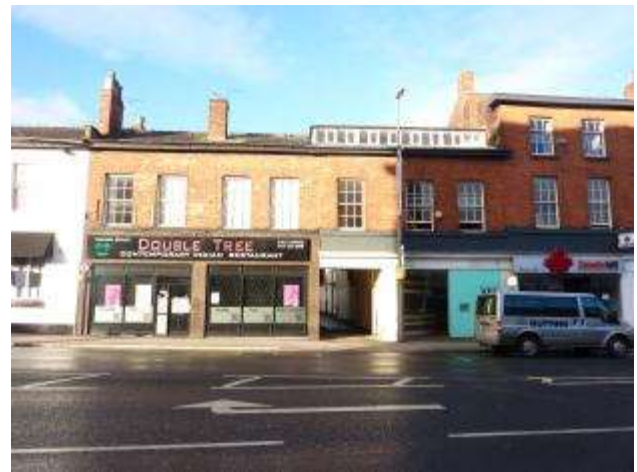
Photograph 9 : Two storey brick buildings on Railway Street
