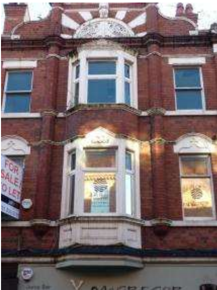
Photograph 12: Decorative gable, pilasters and oriel window
