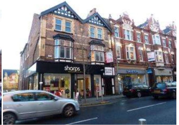
Photograph 11: 25-27 Stamford New Road
