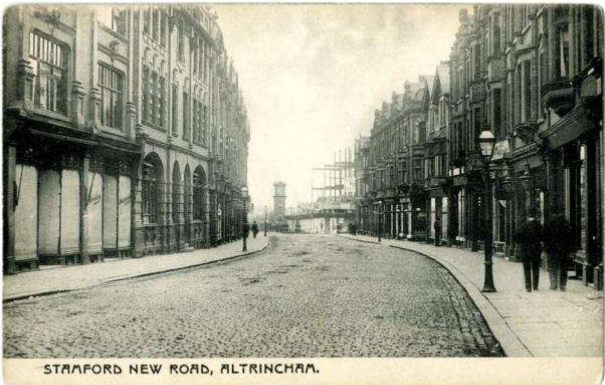
Photograph 2: Stamford New Road, Altrincham with the steel frame of Station Buildings (Stamford House) in the distance, 1905 (Altrincham Area Image Archive)
