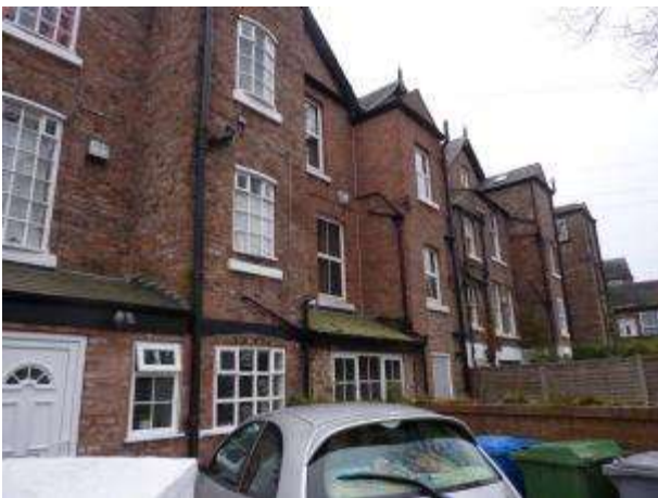
Photograph 34: Rear of Osborne Terrace, 17-23 Hale Road
