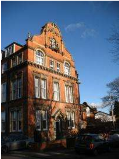
Photograph 50: Telephone Exchange, Woodville Road
