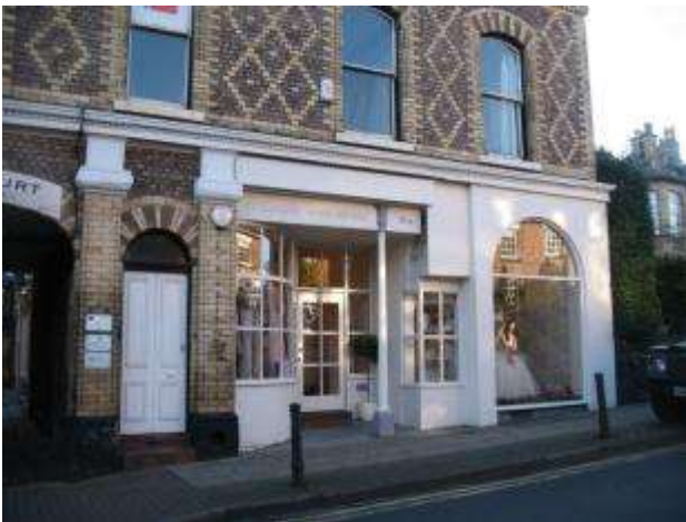
Photograph 20: Modern shop front incorporating pillar, with brick detailing above
