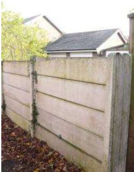
Photograph 42: Intrusive concrete fence on The Narrows
