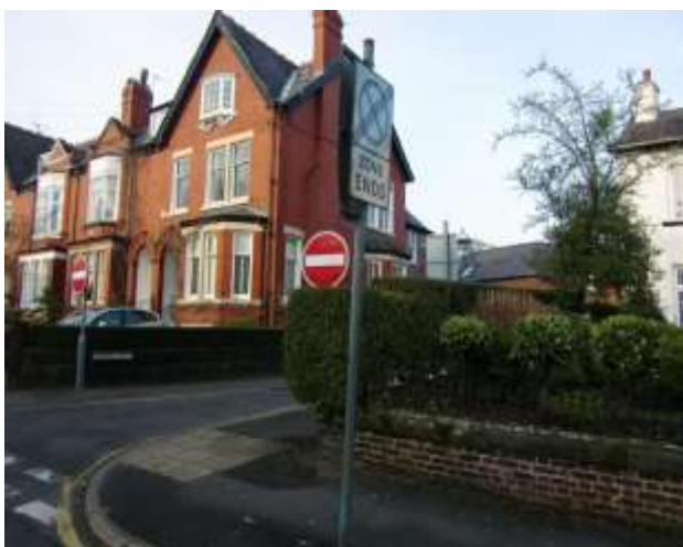
Photograph 44: Excessive parking signage on The Downs
