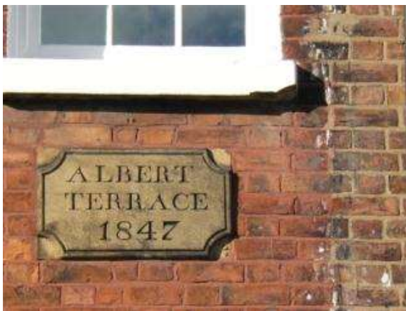
Photograph 4: Stone datestone on Albert Terrace and Flemish bond brickwork, The Downs
