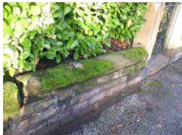
Photograph 11: Stone wall with evidence of historic railings
