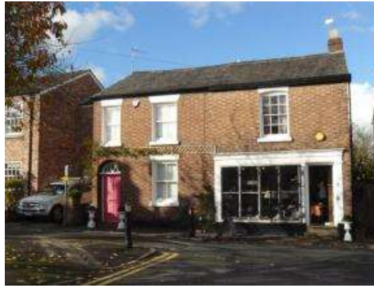
Photograph 7: Worker's housing on New Street and shop front with original features
