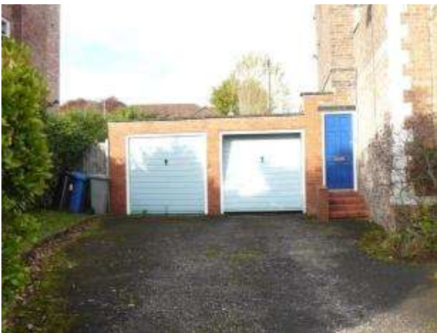
Photograph 40: Intrusive garage/hard standing on Lyme Grove (wide opening not visible)
