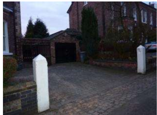
Photograph 41: Lyme Grove garage with traditional form and materials but negative impact on streetscene of wide opening and painted stone gateposts
