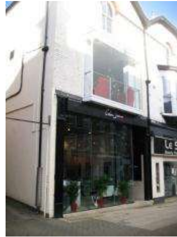
Photograph 39: Inappropriate first floor window
