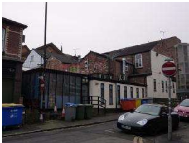
Photograph 35: Rear of 19-23 Ashley Road
