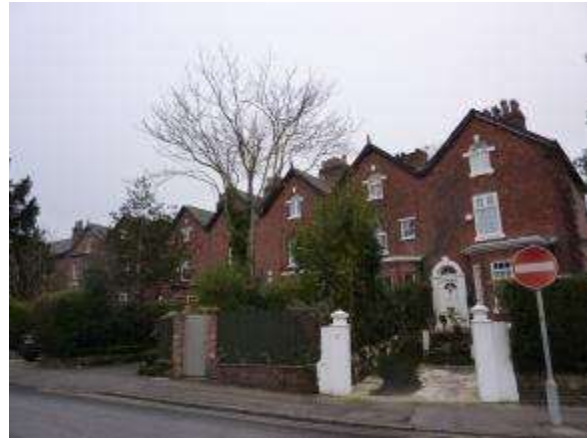
Photograph 49: Removal and alteration of traditional front boundary treatments on Hale Road
