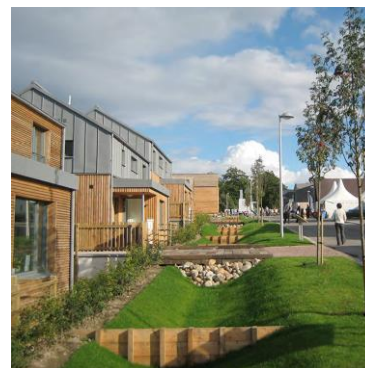
Photograph 40 - Example of a Swale
