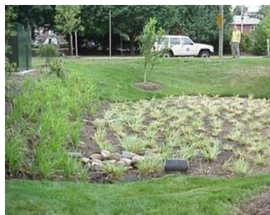
Photograph 38 - Example Bio-Retention Area
