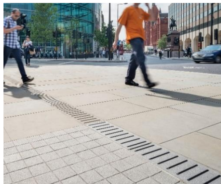
Photograph 45 - Example of a Channel Drain
