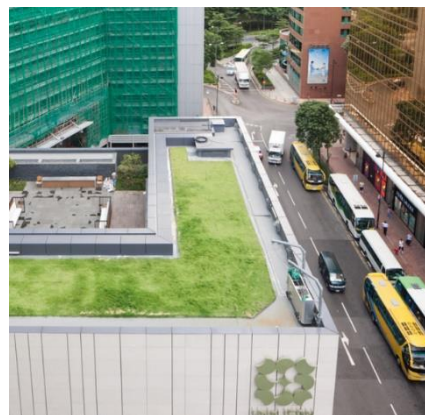
Photograph 46 - Example of a Green Roof
