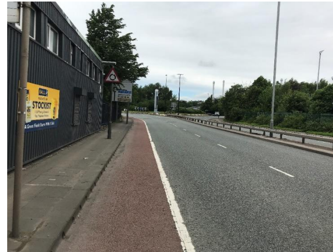
Photograph 5 - The narrow cycle lane on Centenary Way does not provide adequate infrastructure with existing traffic volumes.
