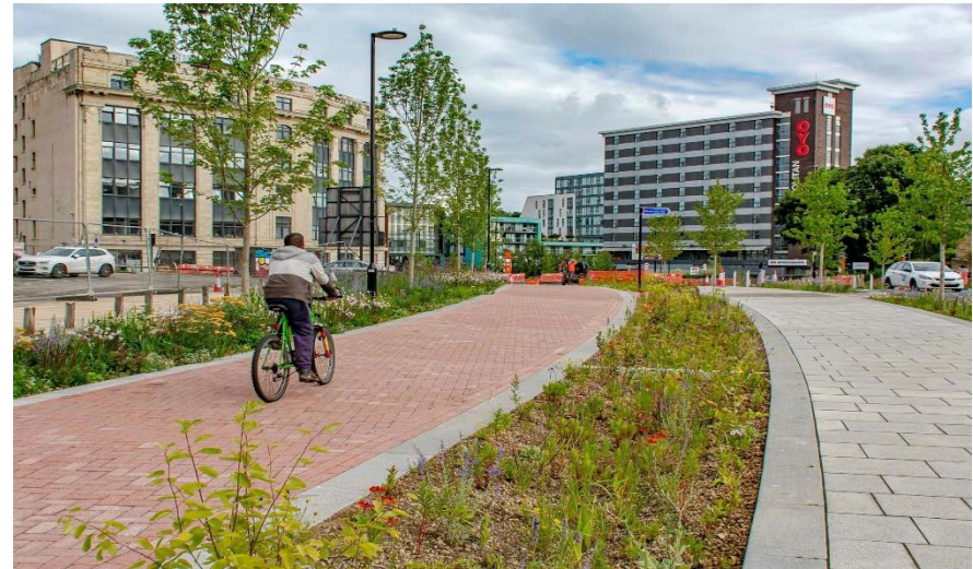
Photograph 37 - Example of rain gardens integrated with active travel infrastructure
