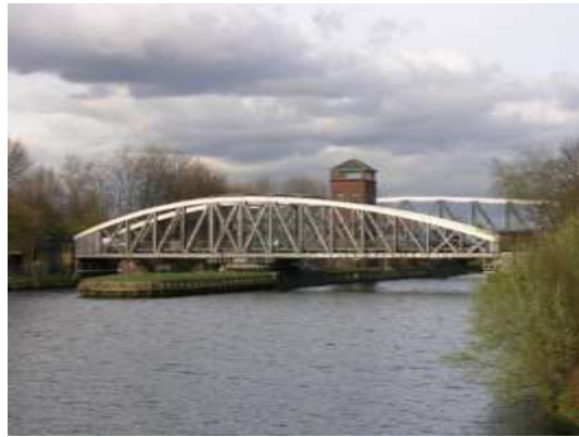
Barton Road Bridge (Wikimedia Commons)
