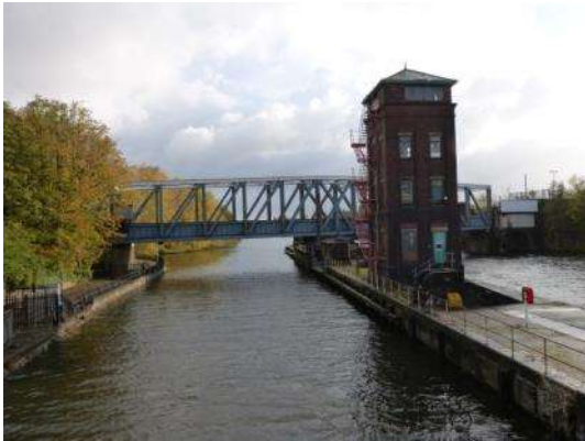
View of Aqueduct and Control Tower from Bridge
