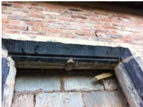
Painted stone window surround, with evidence of former central mullion
