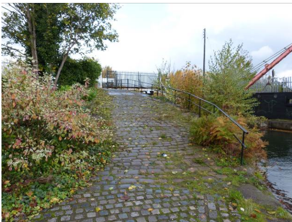
The municipal handrail along the Bridgewater Canal, with the safety fence on the far right
