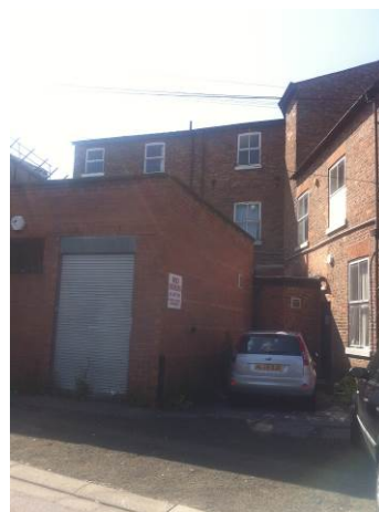
Incongruous infill in The Causeway, which obscures the historic rear elevation fenestration
