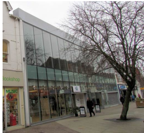
Nos. 74-84 George Street, incongruous for its design as well as its scale and massing
