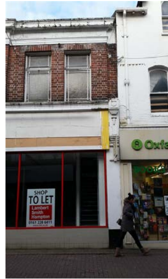
A modern fascia at No. 88 George Street which is notably larger than the historic corbel
