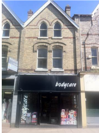
No. 99 George Street, with its original windows
